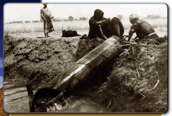
An Archimedes screw being used to irrigate crops on the Nile delta. The device works as a hydraulic screw to raise water from a lower level. J.W. Thomas/Hulton Archive/Getty Images
