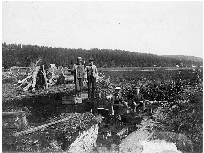
Figure 5.13. The 1908–1919 excavations of the Alvastra pile construction in Sweden.
