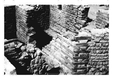
91 Detail of a house at Narmouthis (Medinet Madi). An unusual feature of construction; timber strengthening the angle of the walls.
