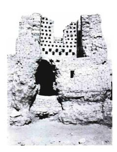
61 Karanis, dovecote tower. The larger dovecores at Karanis were presumably run as commercial ventures or were connected with large estates. This example is a single nesting tower surrounded by singlestorey rooms and courtyards on all sides, covering an area of 12.5 × 10.8 m. The actual nests are wheel-made earthenware pots with rounded bases which were embedded in the dovecote walls.
