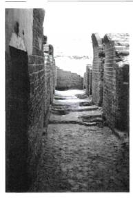
92 A passageway at Karanis. A passage with an arched ceiling which ran between two parts of a large granary. The courses of the bricks are marked by a white lime wash.
