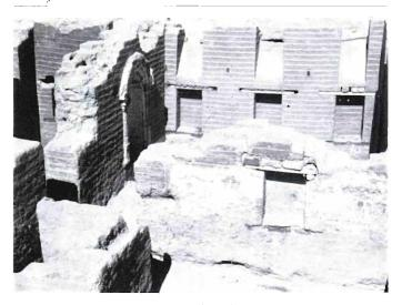
86 A private house at Karanis. A view into a substantial mud-brick house of the Roman period, showing the interior walls with unusually regular brick courses. The niches beneath the windows are surmounted by wooden lintels and will have served as storage cupboards. The wall at the left contains a strine niche which has fluted columns, capitals decorated with scrolls and a shell-shaped top.
