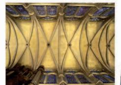
**Ribbed vaulting** helps to support the weight of the high, wide nave ceiling, the highest in France at the time it was built.
