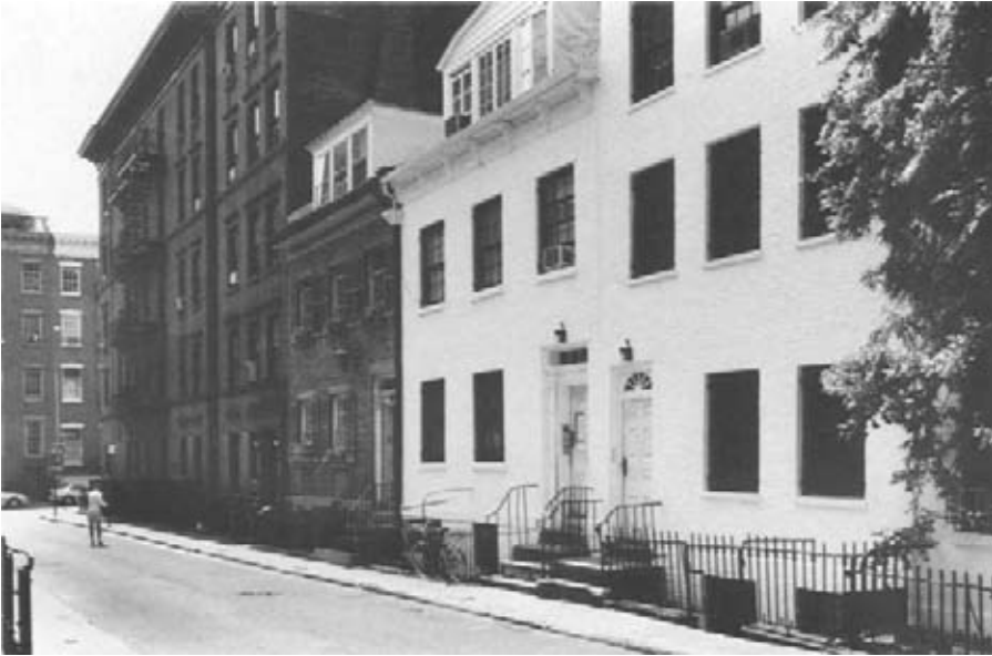
Fig. 8. Modest Artisan-Type Houses, Gay Street, Greenwich Village, New York , buildings, second quarter 19th century; photograph by Dell Upton, July 1998
