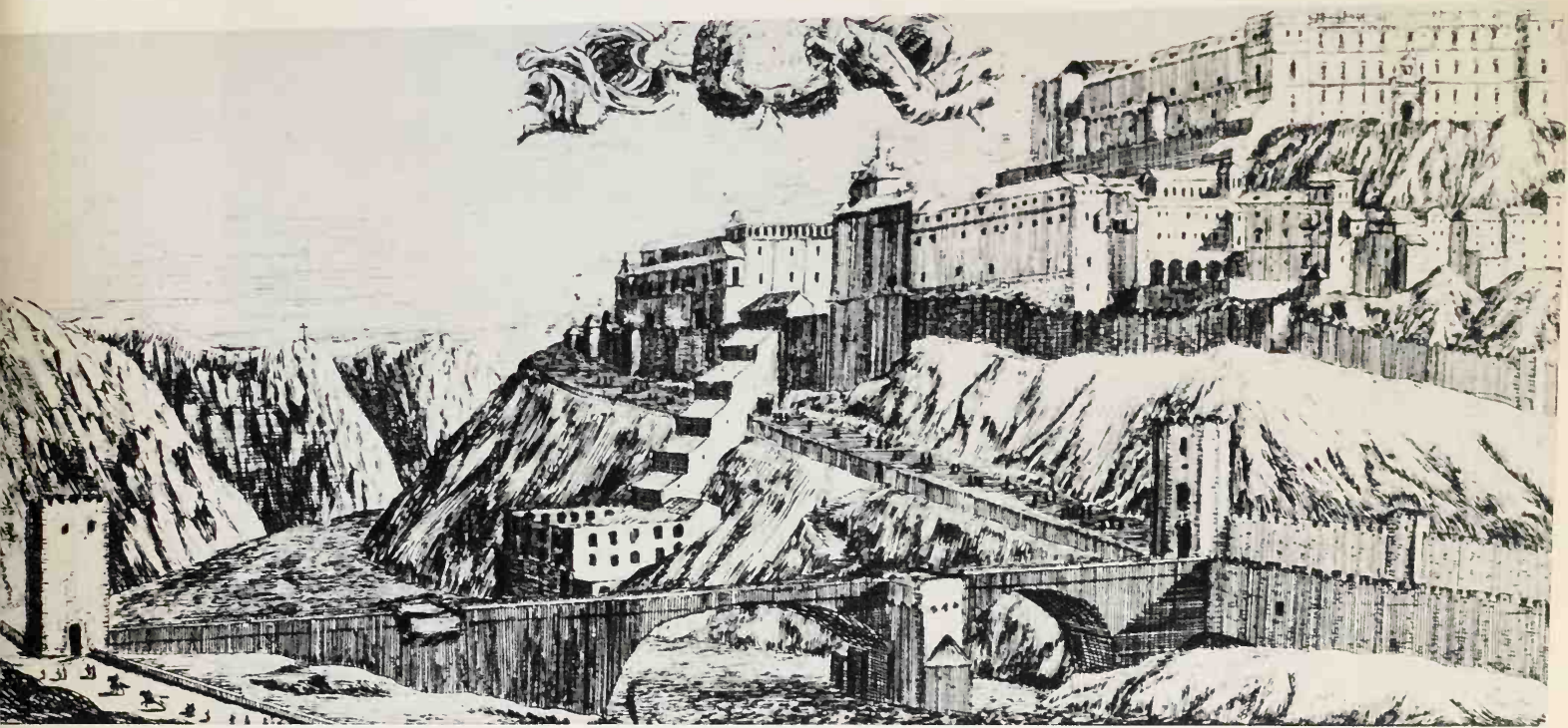
A. Toledo. Bridge and Royal Castle. Engraving by Louis Meunier. Mid-17th C.
