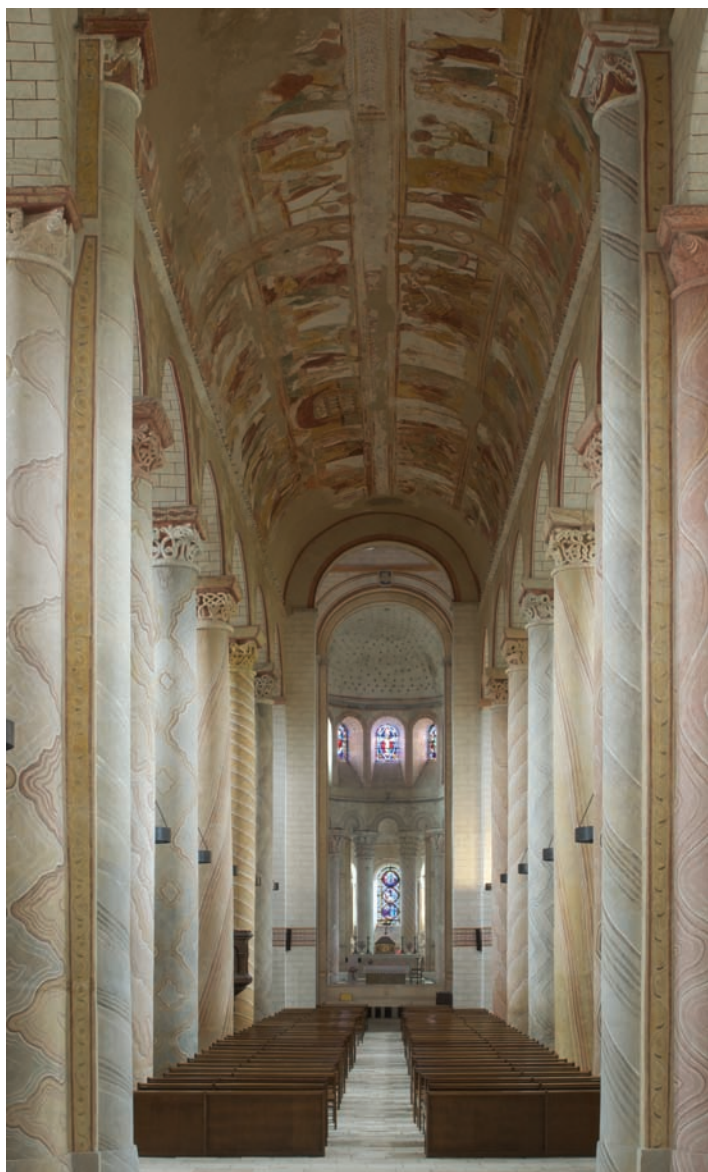
12-17 Nave of the abbey church (looking east) of Saint-Savin, Saint-Savin-sur-Gartempe, France, ca. 1100. ◀
