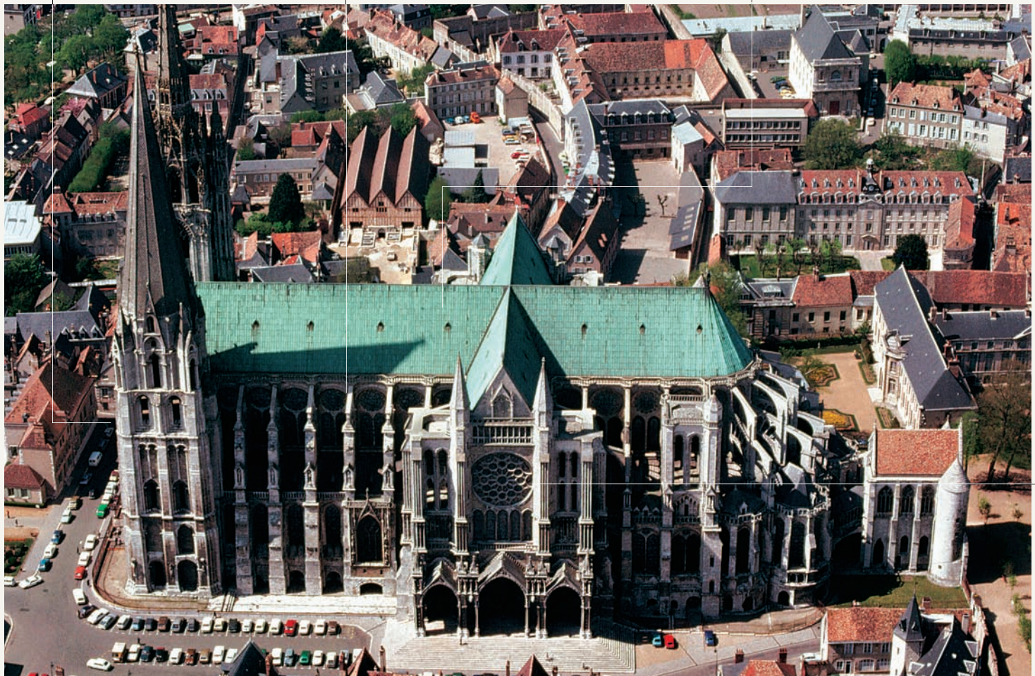
13-1 Aerial view of Chartres Cathedral (looking north), Chartres, France, as rebuilt after 1194. ◀
