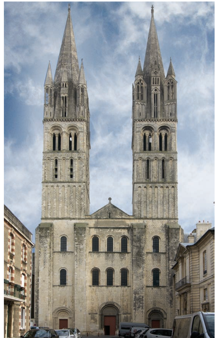
12-30 West facade of Saint-Étienne, Caen, France, begun 1067. ◀
