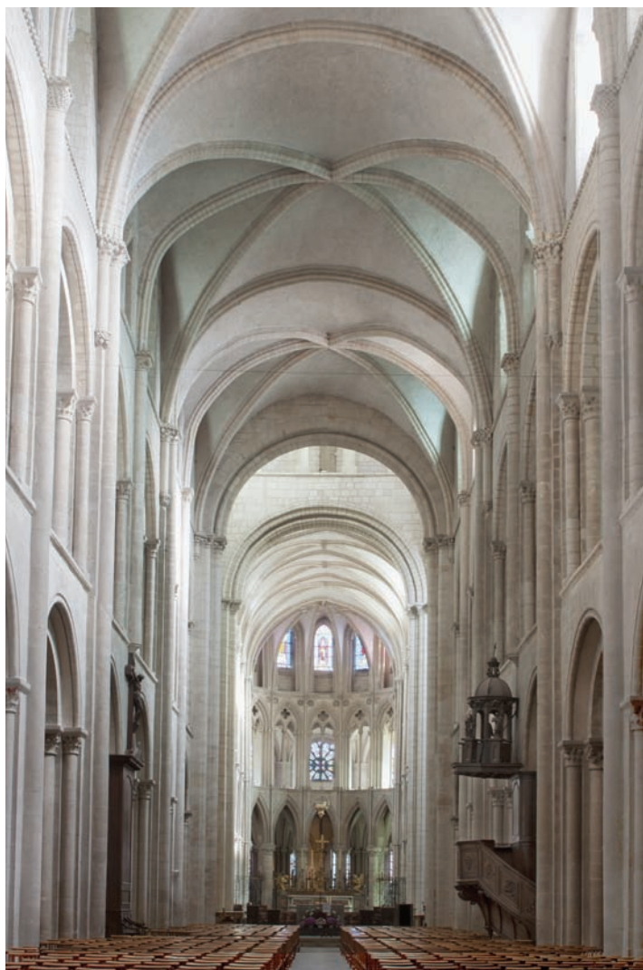
12-31 Interior of Saint-Étienne (looking east), Caen, France, vaulted ca. 1115–1120. ■◀
