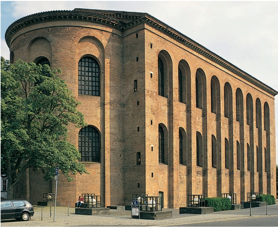
7-79 Exterior of the Aula Palatina (looking southeast), Trier, Germany, early fourth century CE. ■◀
