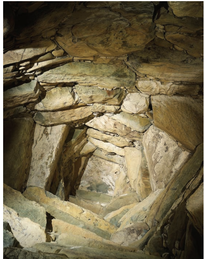
1-18 Corbeled dome of the main chamber in the passage grave, Newgrange, Ireland, ca. 3200–2500 BCE.
