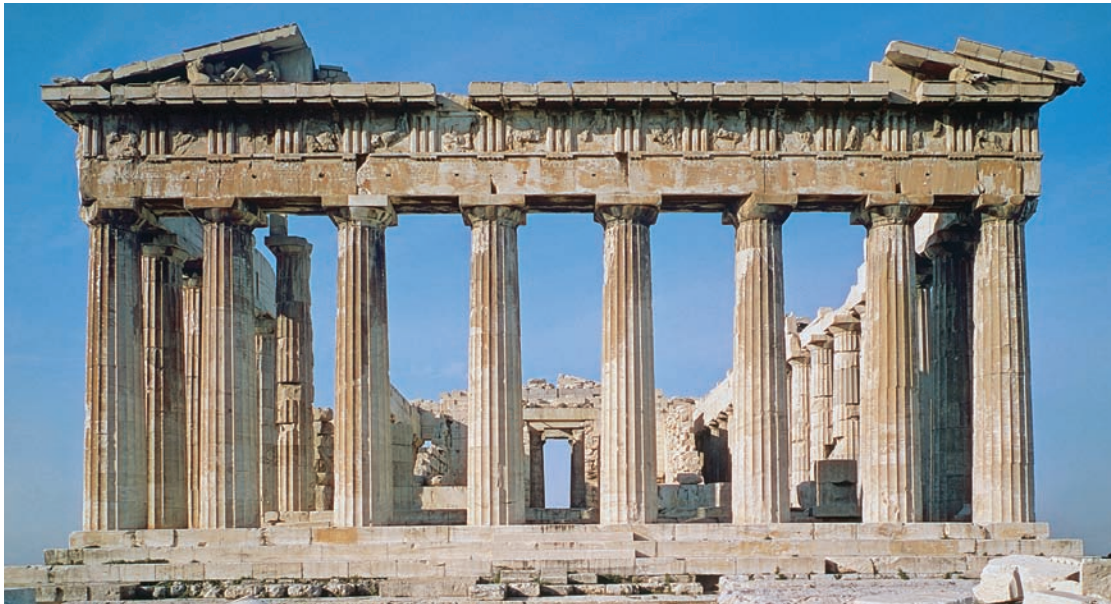
5-44 IKTINOS and KALLIKRATES, east facade of the Parthenon, Acropolis, Athens, Greece, 447–438 BCE.
