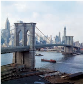
22-46A ROEBLING, Brooklyn Bridge, 1867–1883.
