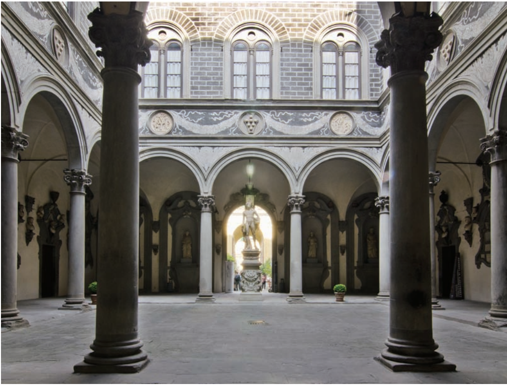
16-38 MICHELOZZO DI BARTOLOMMEO, interior court of the Palazzo Medici-Riccardi (looking west), Florence, Italy, begun 1445. ■◀
