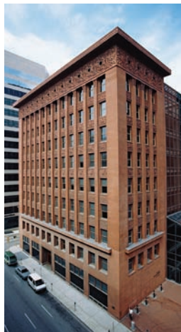
23-40A SULLIVAN, Wainwright Building, St. Louis, 1890–1891.
