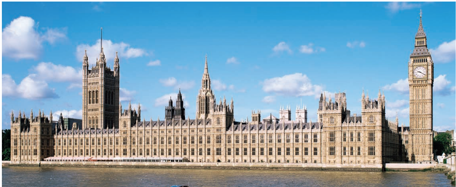
22-43 CHARLES BARRY and AUGUSTUS WELBY NORTHMORE PUGIN, Houses of Parliament, London, England, designed 1835. ◀
