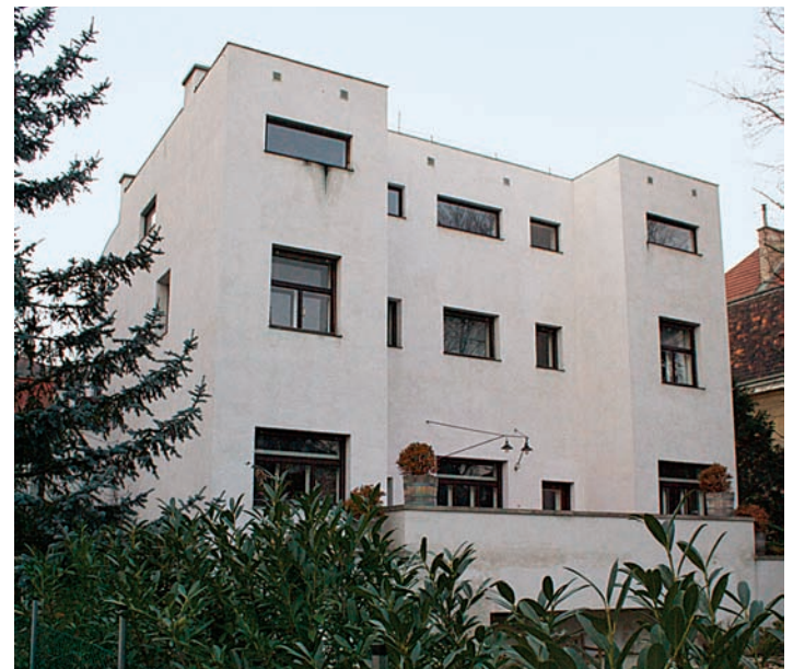
24-33 ADOLF LOOS, garden facade of the Steiner House (looking northwest), Vienna, Austria, 1910.
