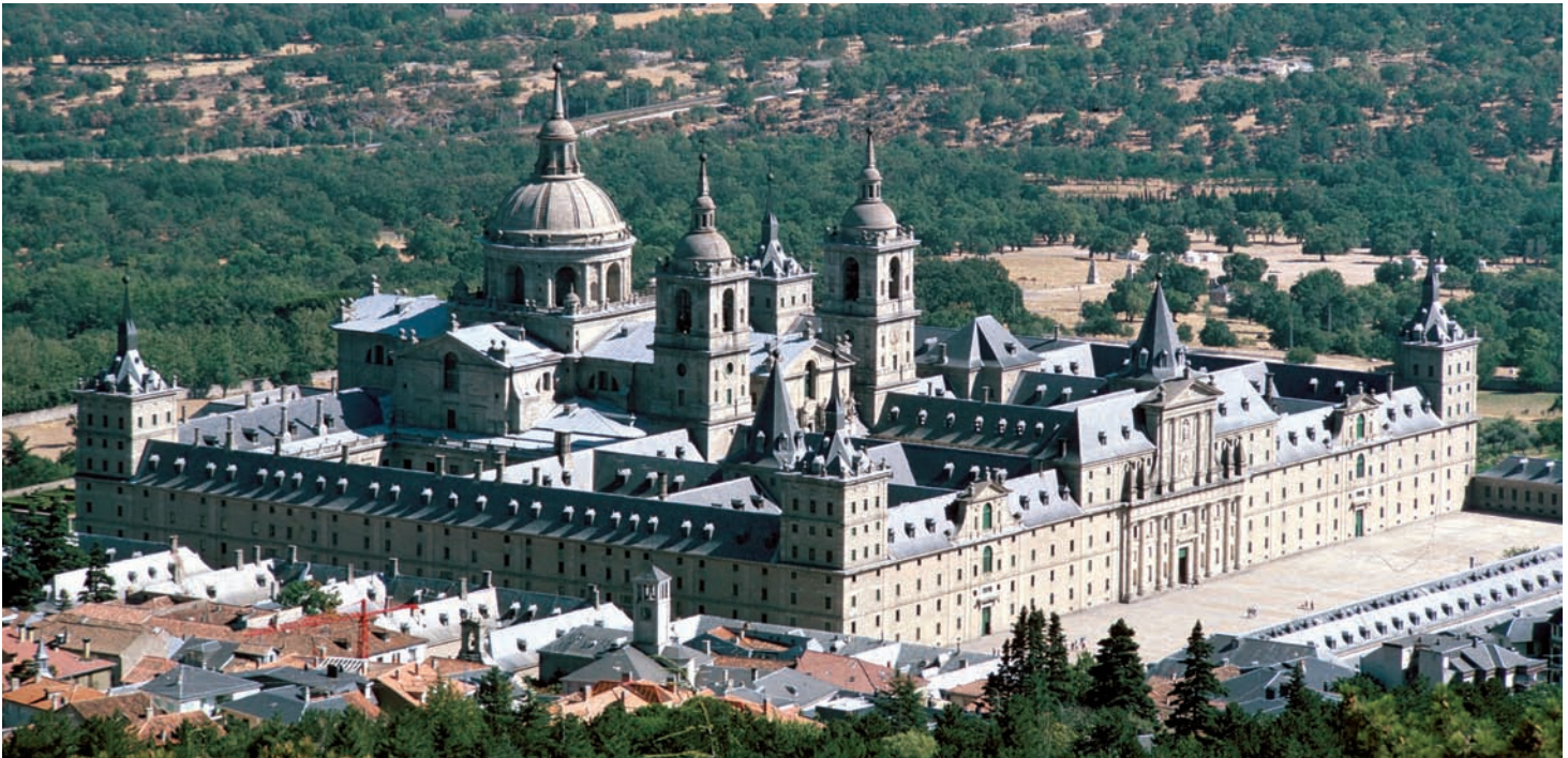
18-24 JUAN DE HERRERA and JUAN BAUTISTA DE TOLEDO, aerial view (looking southeast) of El Escorial, near Madrid, Spain, 1563–1584.
