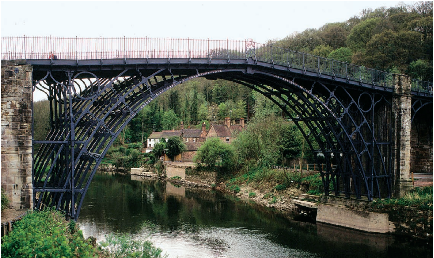
21-12 ABRAHAM DARBY III and THOMAS F. PRITCHARD, iron bridge (looking northwest), Coalbrookdale, England, 1776–1779.
