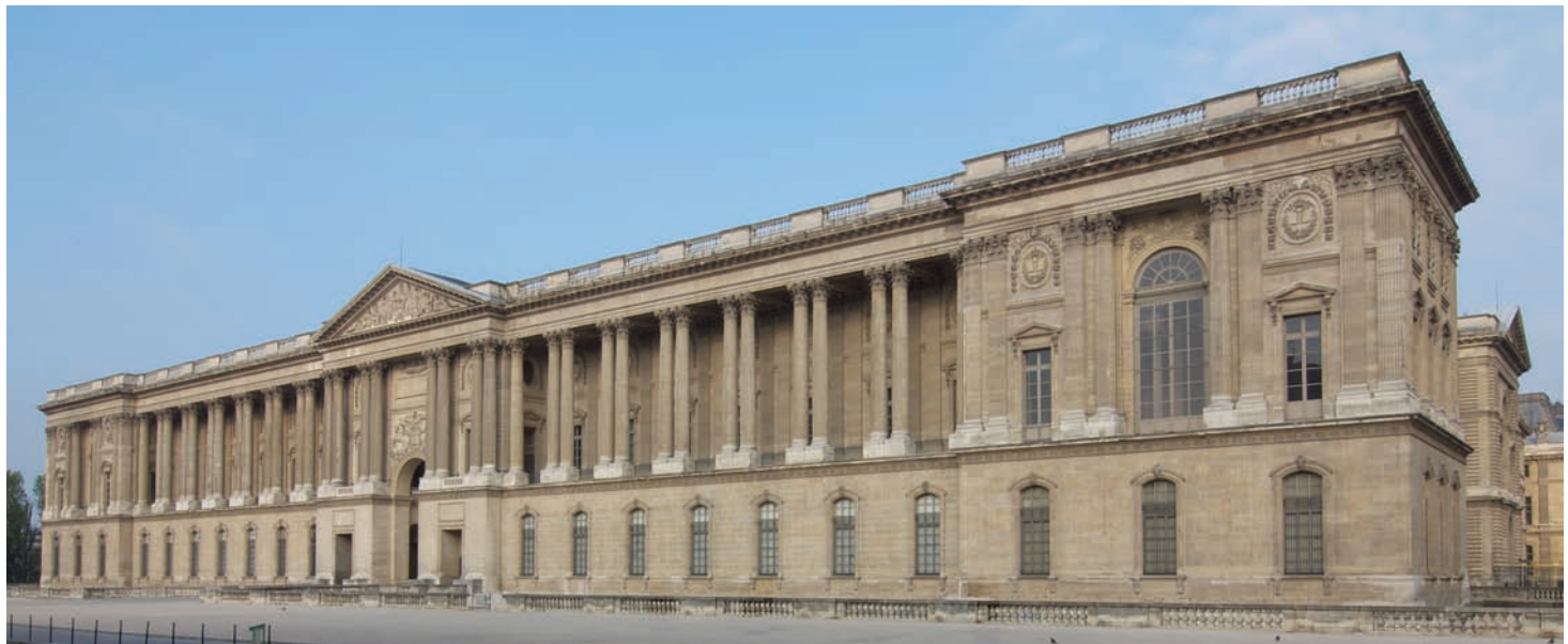
20-25 CLAUDE PERRAULT, LOUIS LE VAU, and CHARLES LE BRUN, east facade of the Louvre (looking southwest), Paris, France, 1667–1670. ■◀
