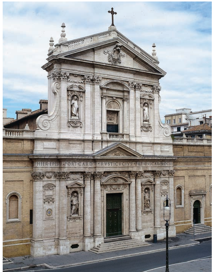
19-2 CARLO MADERNO, facade of Santa Susanna (looking north), Rome, Italy, 1597–1603.
