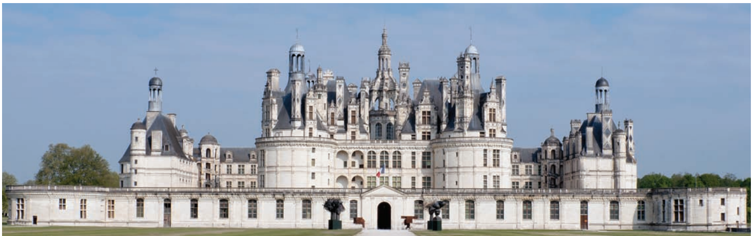
18-13 Château de Chambord (looking northwest), Chambord, France, begun 1519. ■◀
