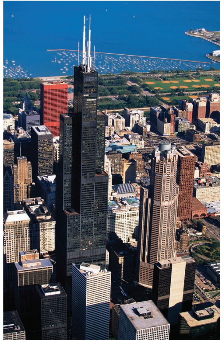
25-44 SKIDMORE, OWINGS & MERRILL, Willis Tower (formerly Sears Tower; looking east), Chicago, 1974. ■◀
