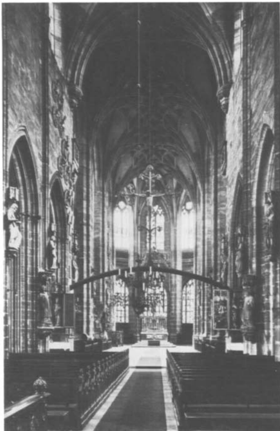
Figure 38 Lorenzkirche: Nave and hall choir, from the west (in 1935)
