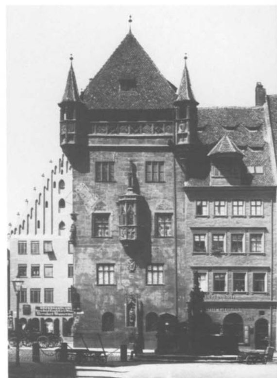
Figure 54 Nassauerhaus, from the east (before 1909)
