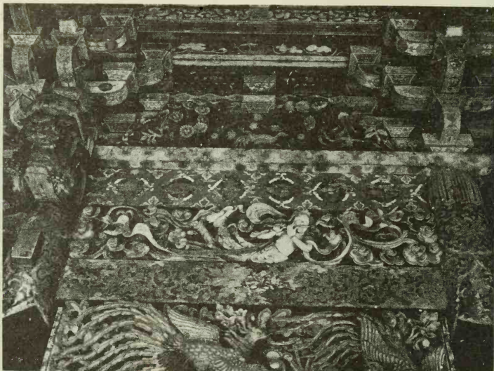
Fig. 167. Interior of Zuihōden Mausoleum Sendai
