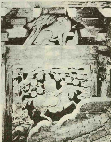
Fig. 136. Open Work of the Kara-mon Gate Nishi-Hongwan-ji, Kyoto
