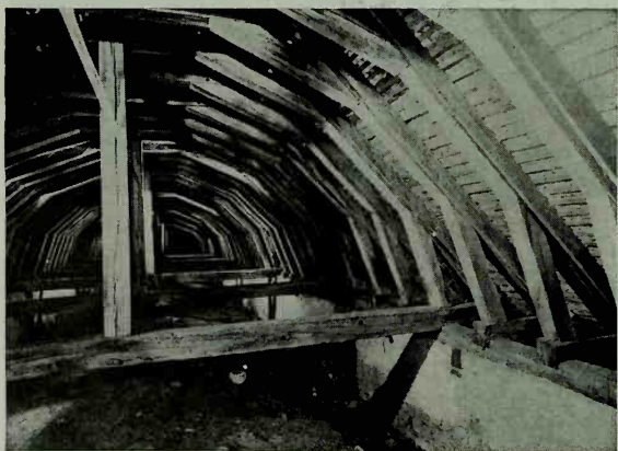
Fig. 7.5 A view underneath the wooden roof superimposed to keep the weather from the tunnel vaulting of a French church of the Romanesque Period.
