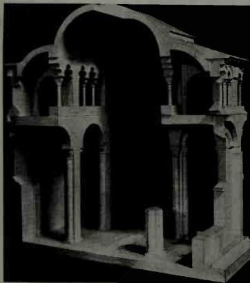
Fig. 7.2 The abutment of a tunnel vault by means of two continuous half-tunnel vaults. From a model of Notre Dame du Port at Clermont-Ferrand.
