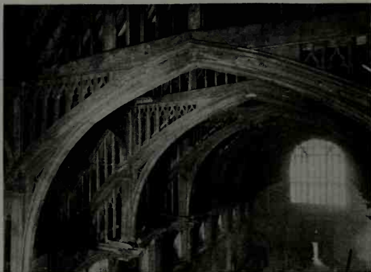
Fig. 12.27 London. Westminster Hall. Hammer-beam roof. 1398. Span: 68 feet.
