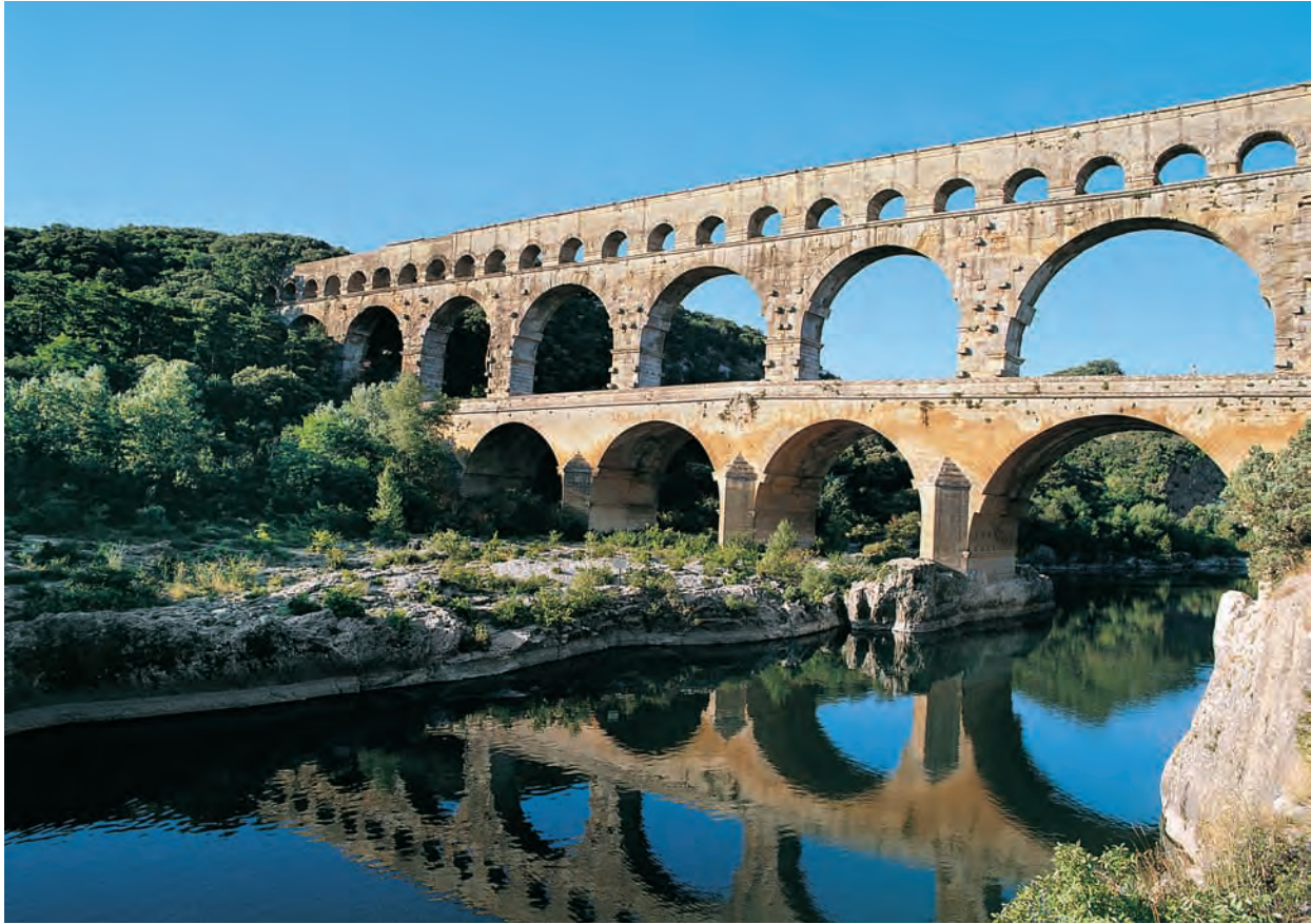
9.14 Pont du Gard, near Nîmes, France, late 1st century B.C. Stone, 854 ft. (260 m) long, 162 ft. (49 m) high. The aqueduct system maintains a constant decline of 1 in 3,000, resulting in a total drop of only 54 feet (16.5 m) over its whole length of 30 miles (48 km).
