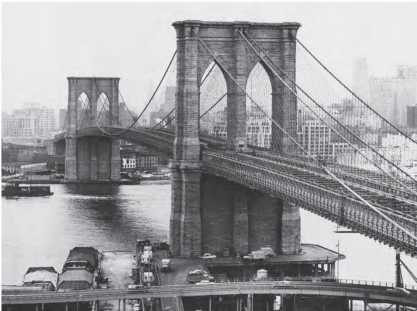
23.20 John A. Roebling and Washington A. Roebling, Brooklyn Bridge, New York, 1869–83. Black-and-white photograph. Stone piers with steel cables, 1,595 ft. (486 m) span. This suspension bridge spanned the East River to connect Manhattan (New York City) and Brooklyn. Like the Crystal Palace, the Brooklyn Bridge was regarded at the time as a work of engineering rather than architecture.
