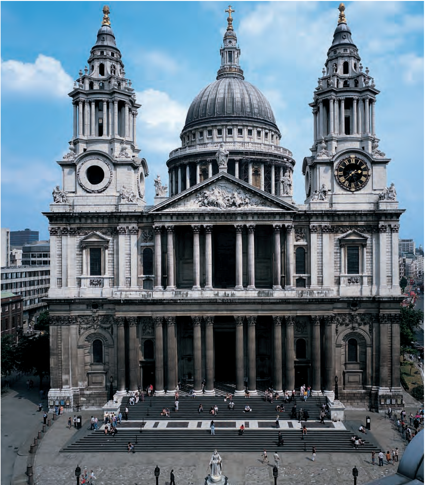
19.12 Christopher Wren, St. Paul's Cathedral, London, western façade, 1675–1710. The dome of St. Paul's is 112 ft. (34.14 m) in diameter and 300 ft. (91.44 m) high, second in size only to St. Peter's in Rome. Even today, the dome dominates the London skyline, although the lower façade is easily visible only from nearby.
