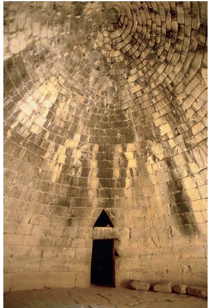
6.18 (Above) Interior of a tholos tomb, showing the entrance lintel and a door to the side chamber. "Treasury of Atreus," Mycenae, 13th century B.C. Diameter of interior 43 ft. (13 m), height 40 ft. (12 m); doorway 17 ft. 8 in. x 8 ft. 10 in. (5.4 x 2.7 m).
