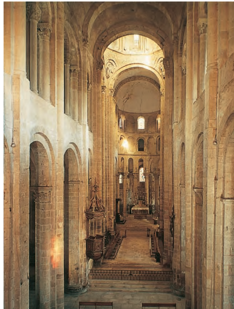
12.4 Tribune and nave vaults, Sainte-Foy, Conques, c. 1050–1120. Romanesque builders solved the problem of supporting the extra weight of the stone by constructing a second-story gallery, or tribune, over the side aisles as an abutment . Structurally, the gallery diverted the thrust from the side walls back onto the piers of the nave. It also provided extra space for pilgrims.
