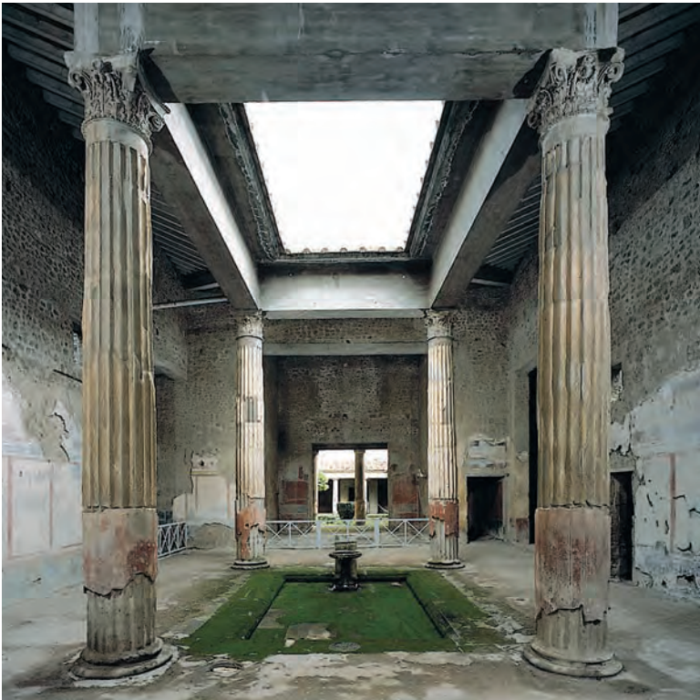
9.3 Atrium and peristyle, House of the Silver Wedding, Pompeii, early 1st century A.D. Standing with our backs to the entrance, we can see the compluvium in the roof, which is supported by four Corinthian columns. The impluvium is in the center of the floor. Visible on the other side of the atrium is the tablinium , probably used for entertaining and for storing family documents and images of ancestors.
