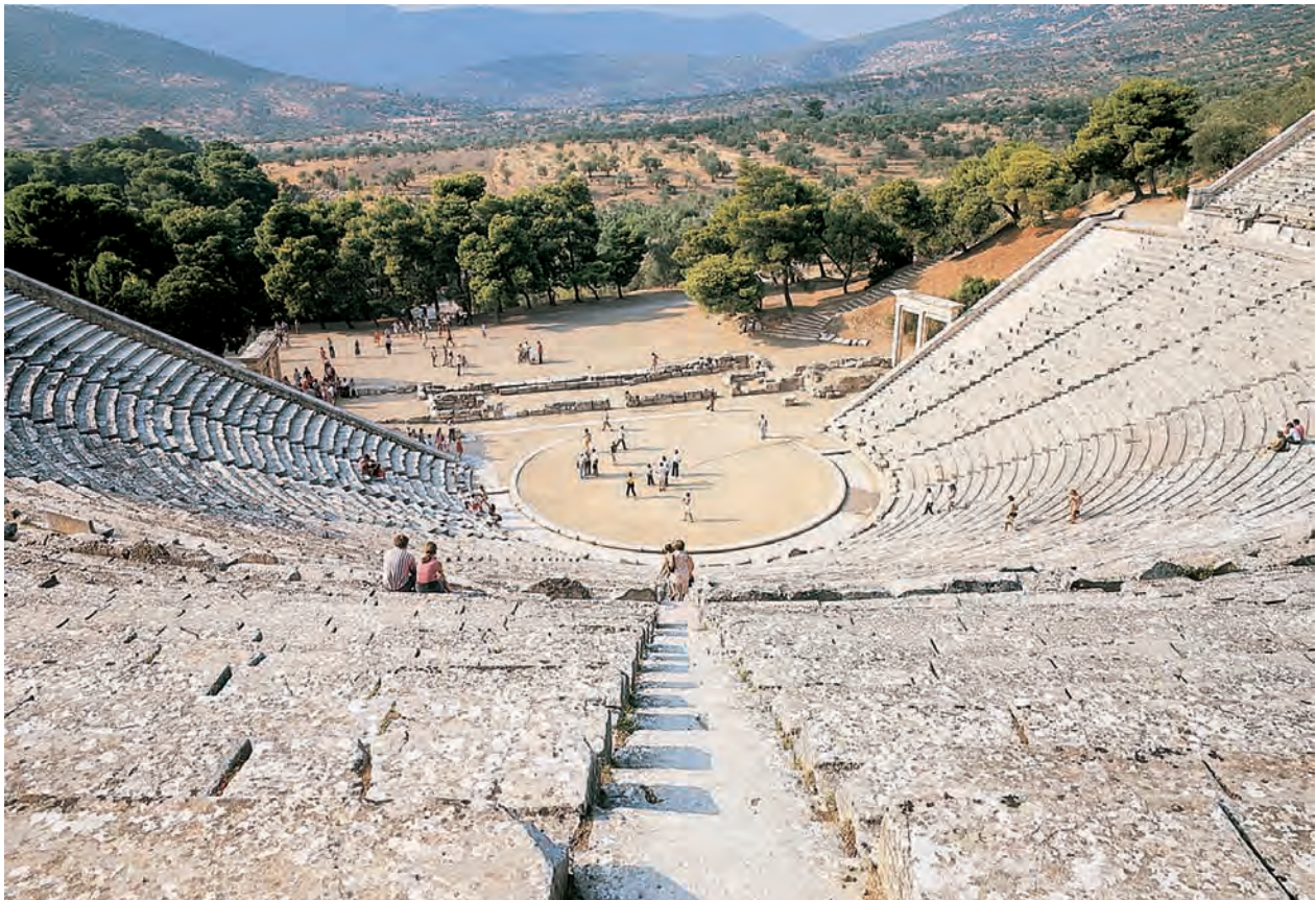
7.32 Theater at Epidauros, c. 350 B.C. Stone, diameter 373 ft. (114 m). Curved rows of stone seats formed an inverted conical space in these impressive structures. Behind the orchestra was the rectangular stone backdrop, or skene (from which the modern English word scene is derived), and actors entered from the sides.
