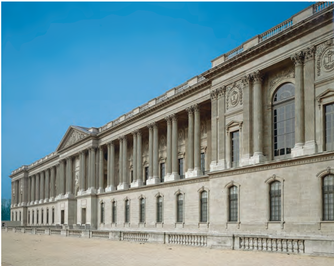
19.8 Claude Perrault, Louis Le Vau, and Charles Le Brun, east façade of the Louvre, Paris, 1667–70. Paired two-story columns separate the windows and are linked by a continuous entablature. The flat roof is hidden by a surrounding balustrade, which accents the horizontality of the building. The central pavilion, resembling a Roman temple front, is crowned by a pediment, which is echoed by the small individual pediments above the windows. The main floor rests on a ground floor presented as a podium . It is lightly rusticated —the blocks of masonry have roughened surfaces and sunken joints.
