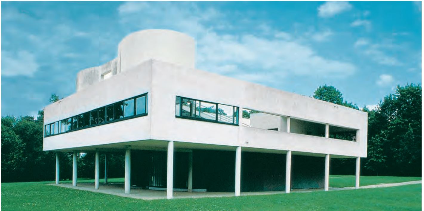
27.27 Le Corbusier, Villa Savoye, Poissy-sur-Seine, France, 1928–30. Le Corbusier believed that houses should be mass-produced. To this end, he reduced architectural components to simple forms—concrete slabs for floors, concrete pillars for vertical support, stairs linking the floors, and a flat roof. In Towards a New Architecture (1931), Le Corbusier wrote, “If we eliminate from our hearts and minds all dead concepts in regard to houses . . . we shall arrive at the ‘House-Machine,’ the mass-production house, healthy (and morally so too) and beautiful in the same way that the working tools and instruments which accompany our existence are beautiful.”
