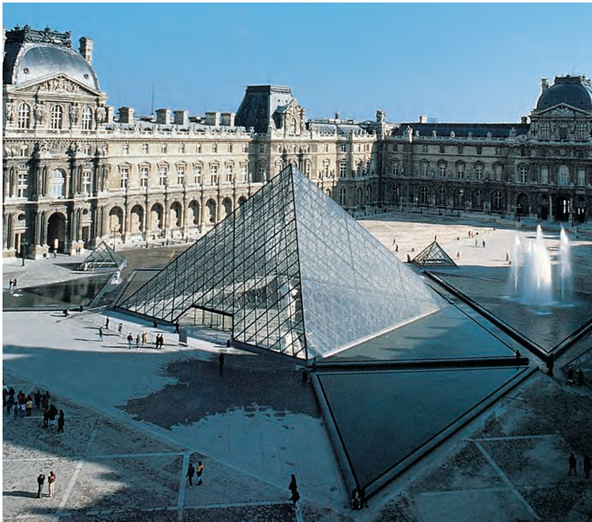
31.11 I. M. Pei, Louvre Pyramid, Paris, 1988. The pyramid is 65 ft. (19.80 m) high at its apex and 108 ft. (32.90 m) wide; it contains 105 tons (107,000 kg) of glass.
