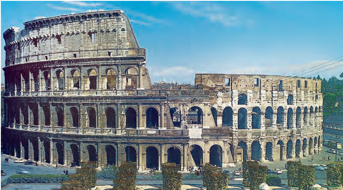
9.12 Side view of the Colosseum, Rome, c. A.D. 72–80. Concrete, travertine, tufa, brick, and marble, approx. 615 × 510 ft. (187.5 × 155.5 m). The term colosseum comes from a colossal statue of Nero. Construction of the Colosseum started c. A.D. 72 under the emperor Vespasian, who had come to power in A.D. 69. It was inaugurated in A.D. 80, a year after his death. More than 50,000 spectators proceeded along corridors and stairways through numbered gates to their seats. The concrete foundations were 25 feet (7.6 m) deep. Travertine (much of it dismantled and reused in the Middle Ages) was used for the framework of the piers, and tufa and brick-faced concrete were used for the walls between the piers. Originally there was marble on the interior, but it has completely disappeared.
