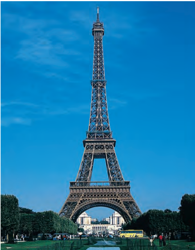
23.21 Alexandre-Gustave Eiffel, Eiffel Tower, Paris, 1887–89. Wrought-iron superstructure on a reinforced concrete base, 984 ft. (300 m) high; 1,052 ft. (320 m) including television mast. The Eiffel Tower was so controversial that a petition demanding its demolition was circulated. When the Exposition ended in 1909, the tower was saved because of its value as a radio antenna. Its original height, before the addition of a television mast, was twice that of the dome of St. Peter's or the Great Pyramid at Giza. Until the Empire State Building was built in New York in 1932, the Eiffel Tower was the highest man-made structure in the world.
