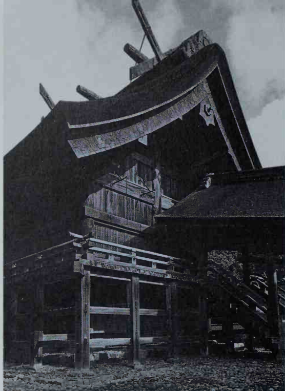
15 Izumo Taisha Shintō shrine (rebuilt 1744), showing covered stairway (and Main Sanctuary with deep thatch).
