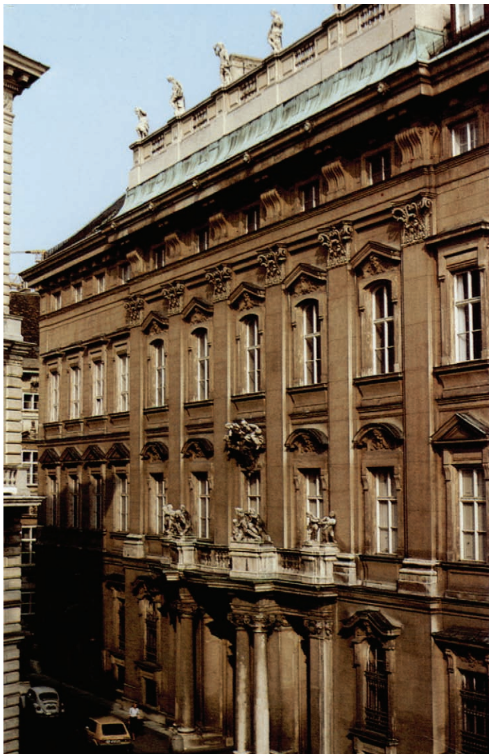
Fig. 9 The Liechtenstein City Palace in Vienna, designed by Domenico Martinelli (1650–1718) and built in 1689–1700, was the princely family’s main residence until 1938.
