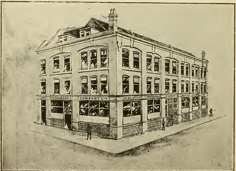
CHURCH STREET AND NICHOL STREET WAREHOUSE.
