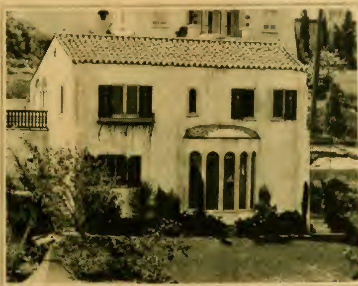
Valentino's house, high in Beverly Hills, is cracking and slipping
