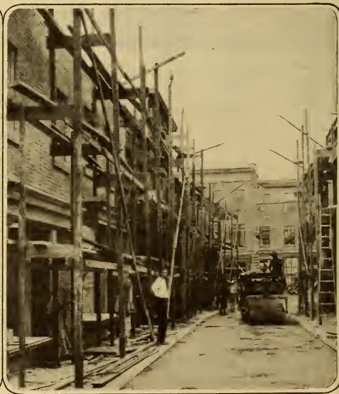
Scaffolding constructed from material salvaged from the scrap heap.
