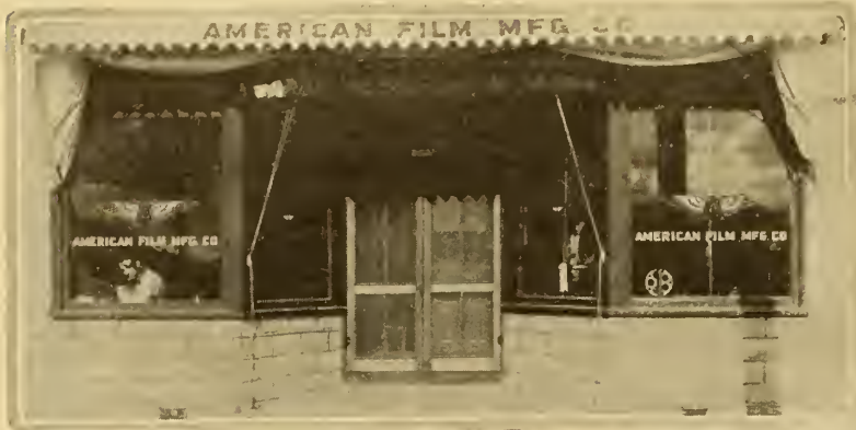
Facade of the "Flying A" Studio in Santa Barbara as it was five years ago when the American Company settled there. The Studio was built in the corner of an ostrich farm which has given way to commercial improvements.
