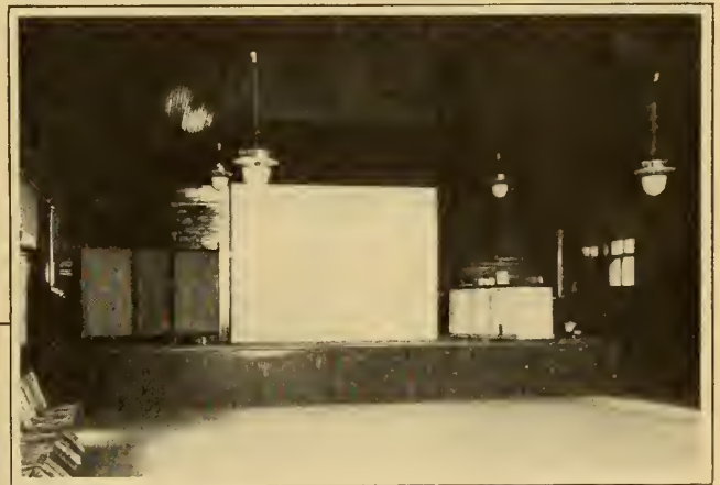
An interior view of Amusement Hall.
