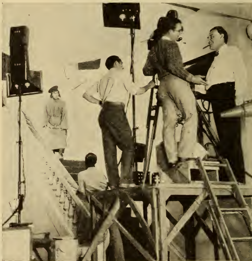
Another one of those things that seem so simple on the screen. Benjamin Christiansen had this elaborate contraption built so that he might get a good shot of Lon Chaney starting downstairs. The title of the newest Chaney picture—a Russian story—has been changed from "Terror" to "Mockery." It's all right with us
