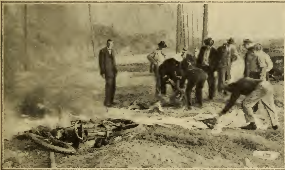
"Speed" failed to pull his 'chute and crashed to the ground. He's in the hospital now, figuring out how he can make the leap in a Ford coupe. There's your true stunt man!
