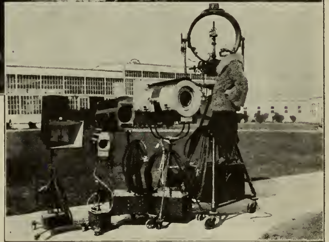
Here are types of the lights used. From left to right they are the Creco Broad; the 35-ampere "baby spot"; the 70-ampere spot; the 110-ampere spot; and the 120-ampere Sunlight arc. The human light is Carmelita Geraghty
