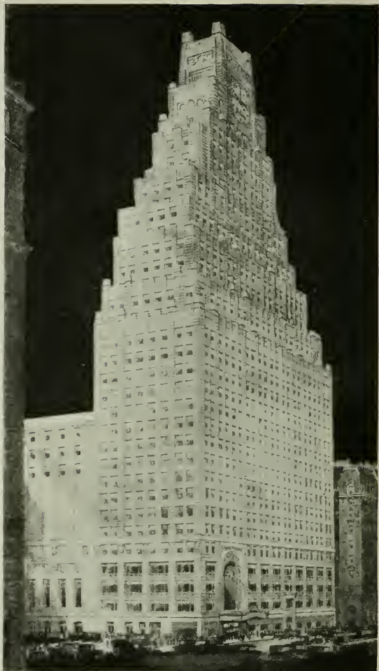
Famous Players' new theater building is destined to become a landmark of New York. It is now being constructed in Times Square, "the crossroads of the world." The base of its thirty-five stories of steel columns rests upon solid rock fifty-two feet below the street level. It will be 450 feet high and is the first great monumental structure erected by the motion picture industry.
