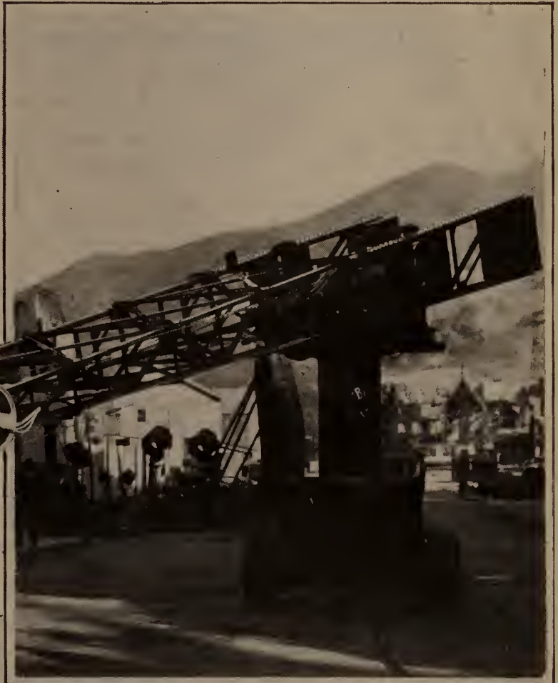
The camera crane lowered to take a shot at a little above street level. Paul Fejos, director of "Broadway," and inventor of the idea of the ingenious crane, is seen on the platform.
