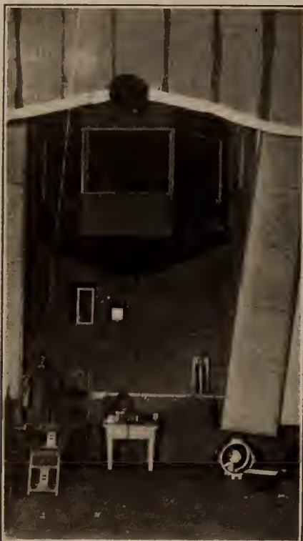
Exterior of monitoring room in Universal's new talkie stage.
