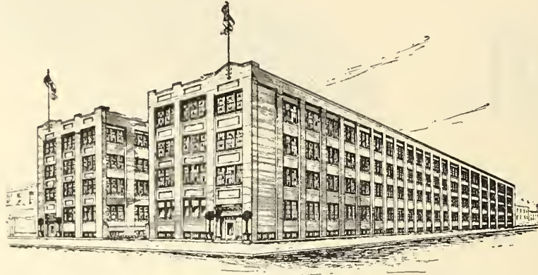
The new factory at St. Thomas, Ontario, now in construction
