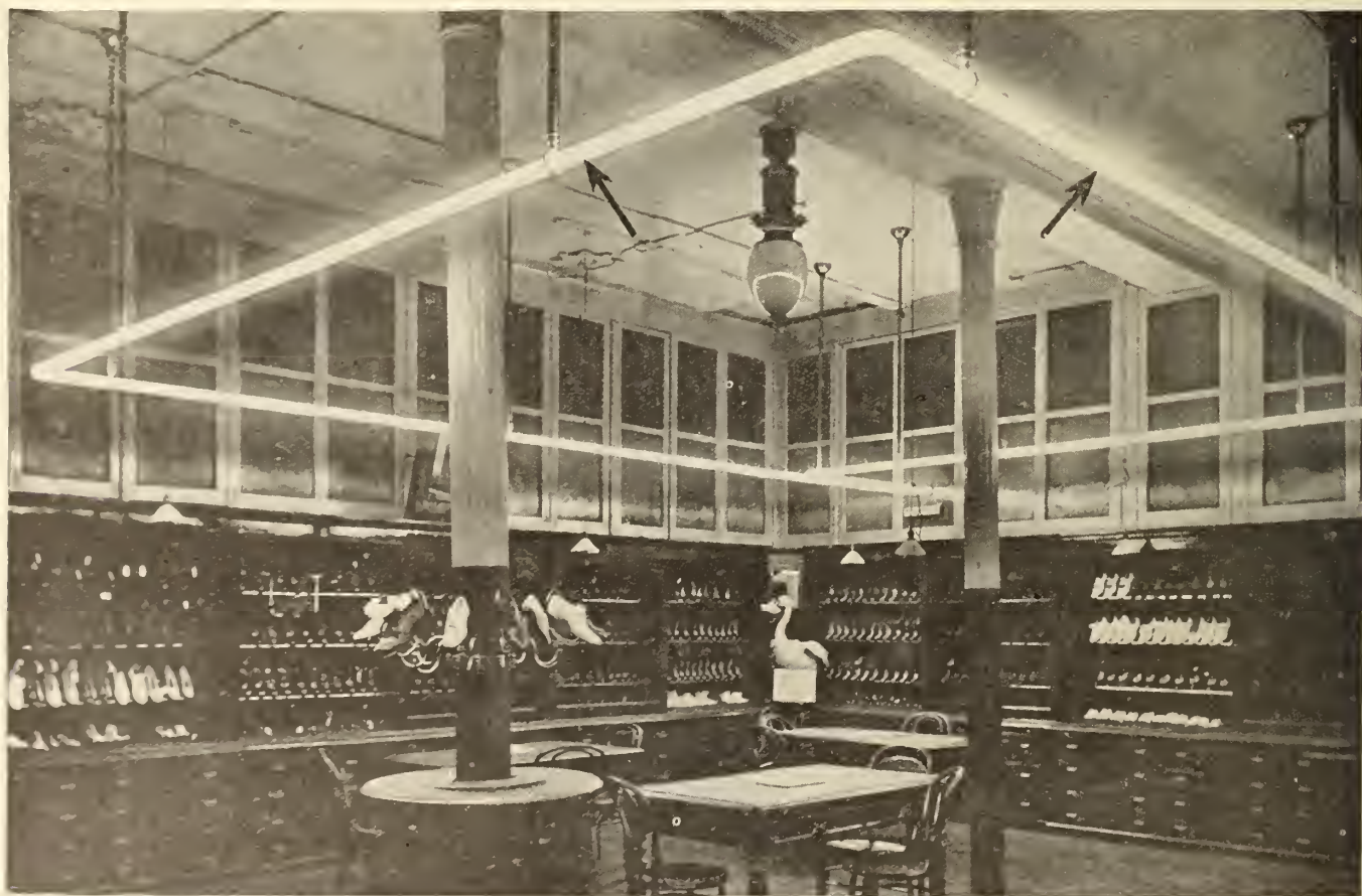
The Continuous Tube: A novel and, as yet, uncommon method of store lighting. The passage of a current of electricity through gases in a vacuum tube produces a soft, diffused but efficient illumination. By the use of the proper gas, a white light can be secured.
