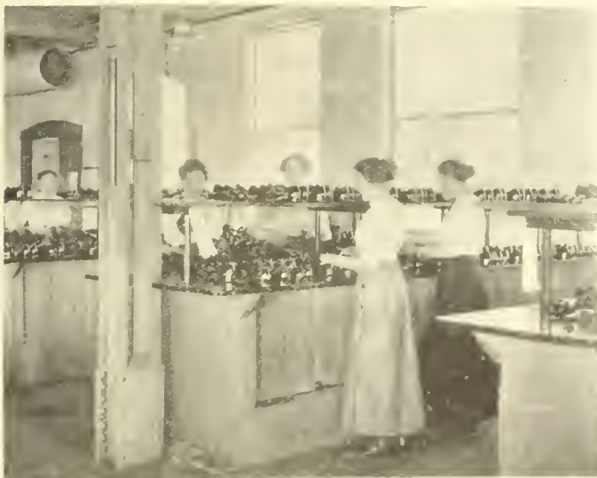
Trimming Shoes after Vulcanization
