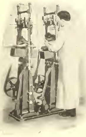
15. Twin Sole Laying Machine
