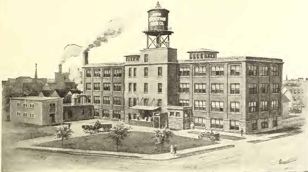
The New Factory of the John Strootman Shoe Co., Buffalo, N. Y.
