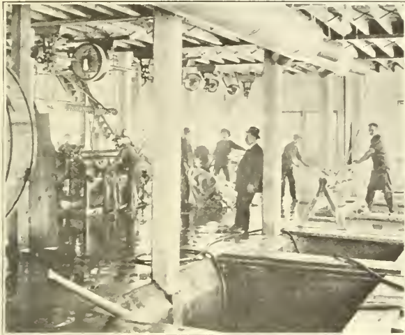
Portion of Tannery, showing vats and revolving drum.
