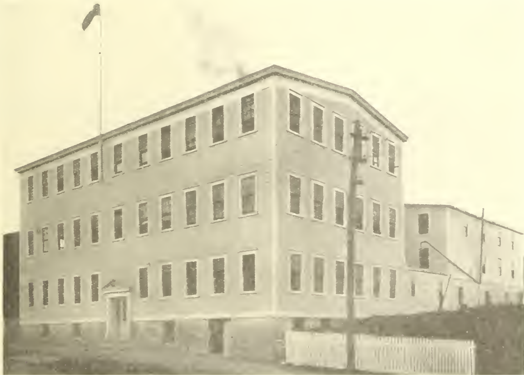
Factory of the Harbor Grace Boot & Shoe Manufacturing Company, Limited, Harbor Grace, Newfoundland
