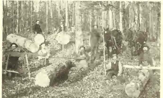
Sawing Timber into "cartwheels." Note saw filer on left.
