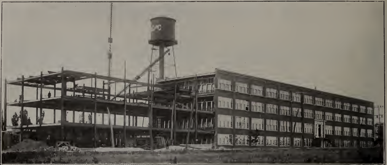
Photographic Cut Showing Completed Fabrication of Steel from Corner
