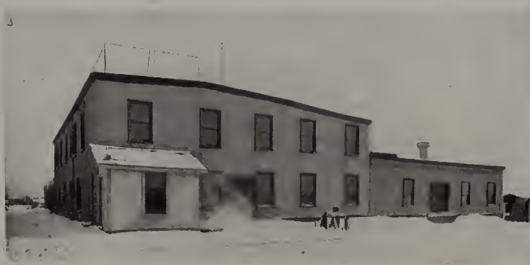
No. 2 Factory, Laing St.
