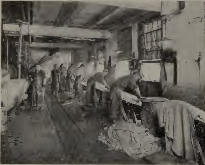
A section of the beam house
