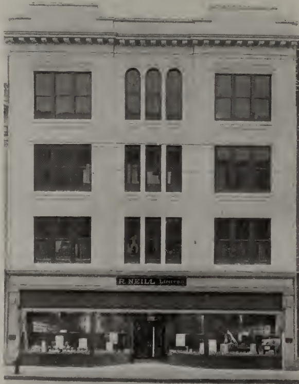
The visitor to Peterboro is instantly attracted by the handsome exterior of the Neill Building
