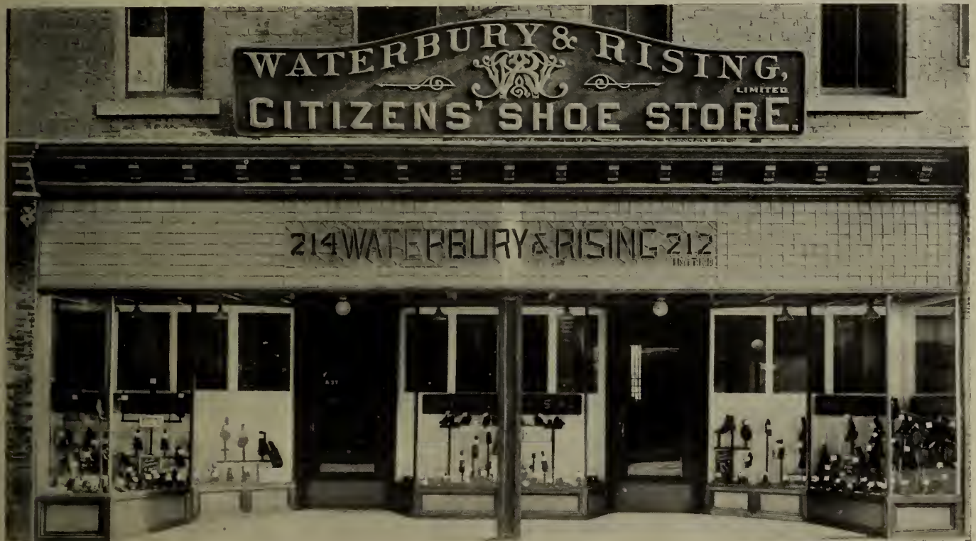
Attractive new store front installed in Union Street store of Waterbury & Rising, St. John, N.B., by Kawneer Manufacturing Company.
