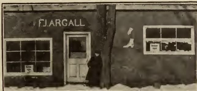
TEMPORARY STORE BUILT AFTER THE FIRE IN THREE RIVERS, QUEBEC, IN 1908
