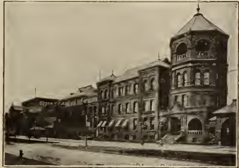
MECHANICS' BUILDING, BOSTON (THE SCENE OF THE SIXTH NATIONAL SHOE AND LEATHER MARKET FAIR).
