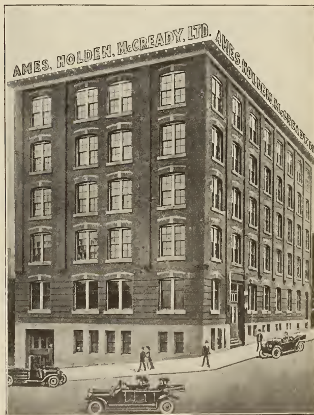
Attractive New Warehouse in St. John
