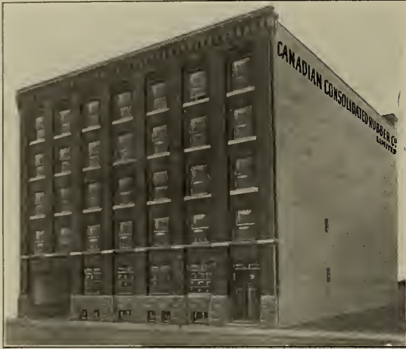
THE NEW CALGARY WAREHOUSE
