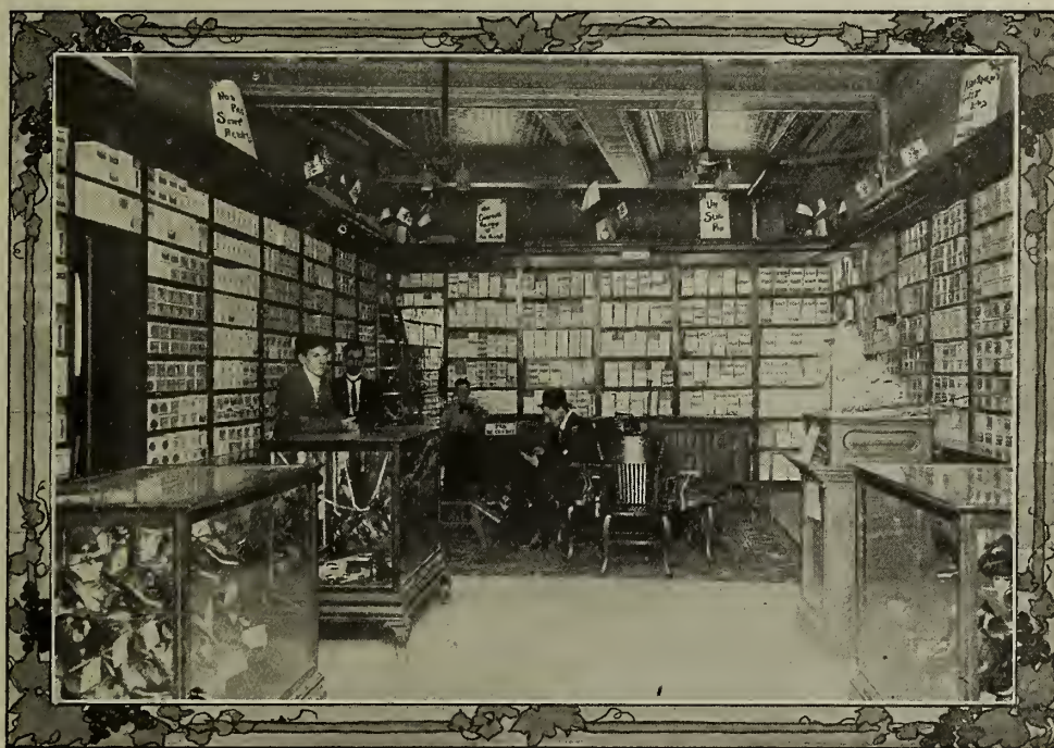
THE INTERIOR OF A. CORBEIL'S STORE AT THREE RIVERS, QUE.
