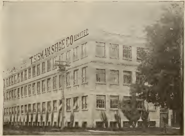
Offices and Factory, Aurora, Ont.
