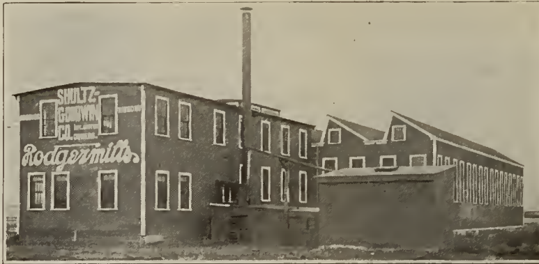
LENGTH OF MILL 175 FEET
