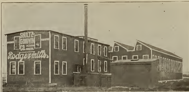
LENGTH OF MILL 175 FEET
