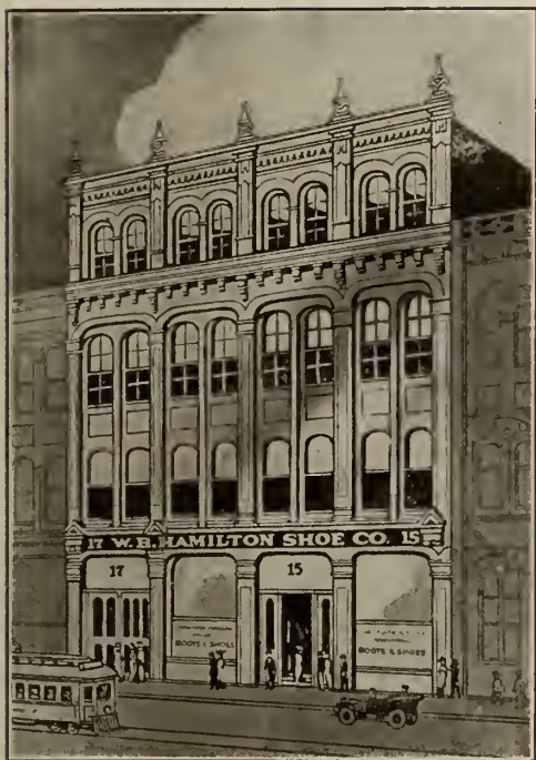
Offices and Warehouse
