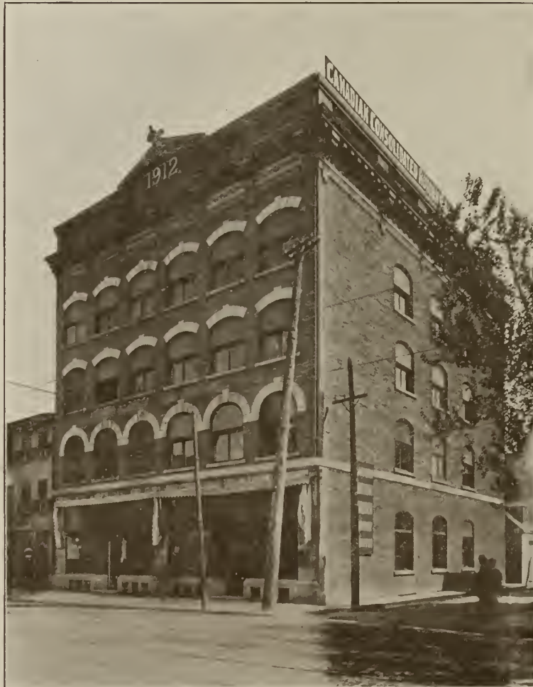
THE BEGIN BUILDING IN WHICH THE QUEBEC BRANCH OF CANADIAN CONSOLIDATED RUBBER CO. IS LOCATED
