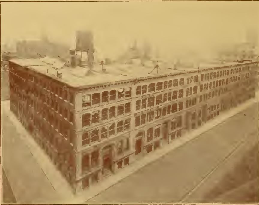
HEAD OFFICE AND FACTORY: VICTORIA SQUARE, MONTREAL
