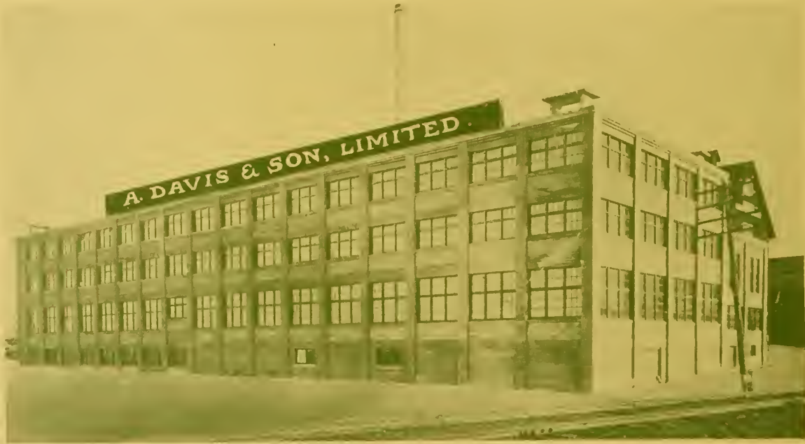
View from the north-west corner. In the rear are the large Concrete Store House, Leach House and Bark Sheds, and also the Boiler and Engine Rooms, of re-inforced Concrete
