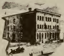
Head Office, Kitchener
