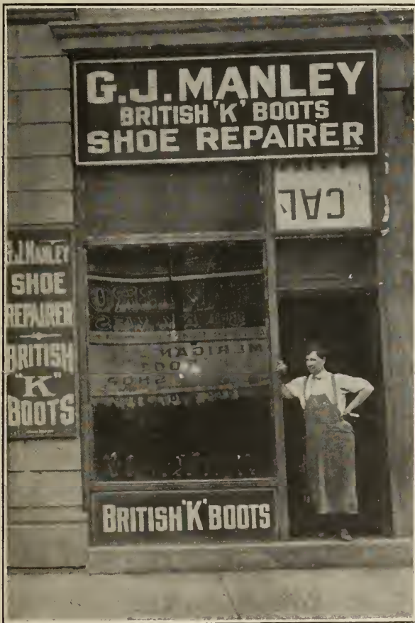
Geo. J. Manley, 8th Avenue, Calgary, Alta., (at door) who has just completed the installation of the latest in shoe repairing Machinery, being a 22 foot Goodyear Repair Outfit, with the new covered in Goodyear Stitcher and a Model S McKay Sewing placed in line so that the whole is operated from one motor. Mr. Manley is an enthusiastic gardener, a great lover of good flowers, and as a fisherman and good sportsman is well-known in Calgary.
