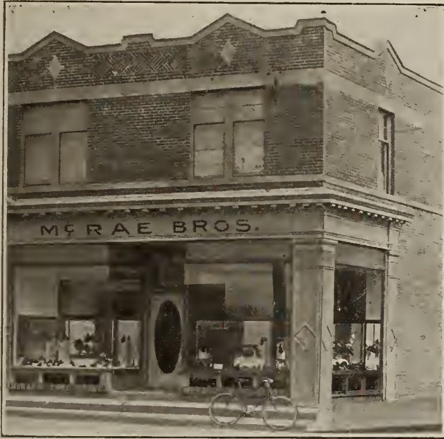
THE ATTRACTIVE HOME OF A PROGRESSIVE SHOE FIRM IN CAMPBELLTON, N.B.
