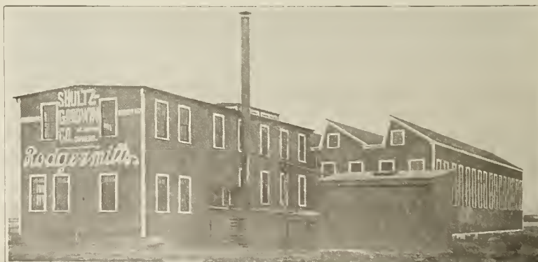
LENGTH OF MILL 175 FEET
