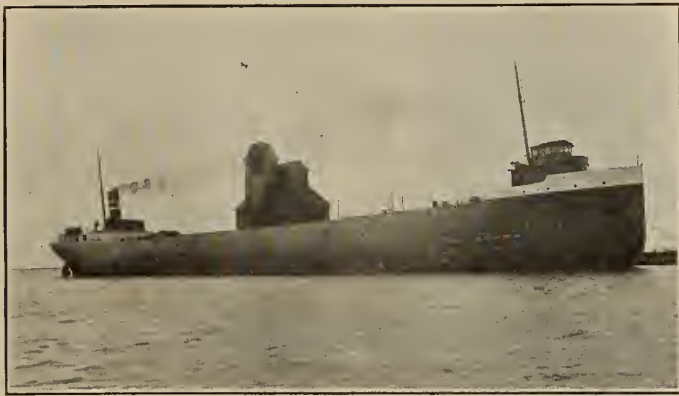
A view of the S.S. Laketon showing new bow.
