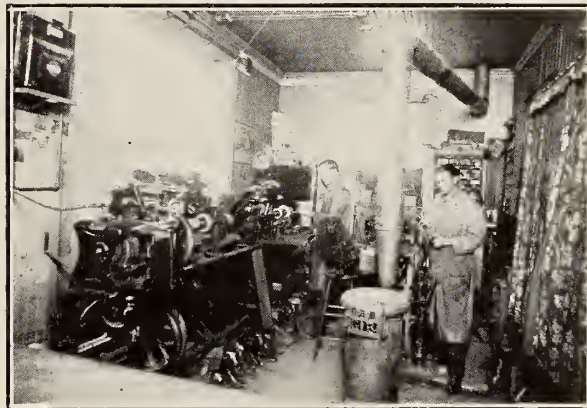
Mr. W. A. Greenslade's Repair Plant, Peterboro
