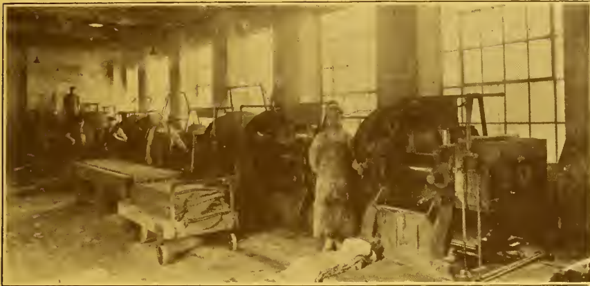
Rubber Washing Room
