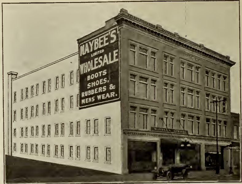
The present splendid wholesale establishment of Maybee's Limited, 121 to 125 High street, west, Moose Jaw, Sask.
