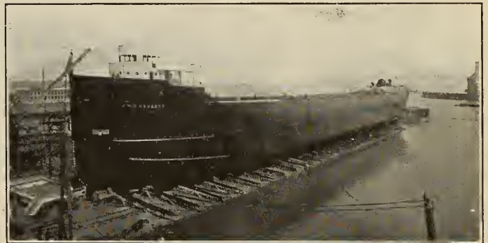
A 11,000 tons Freighter, 550' x 58' x 31' ready to launch.
