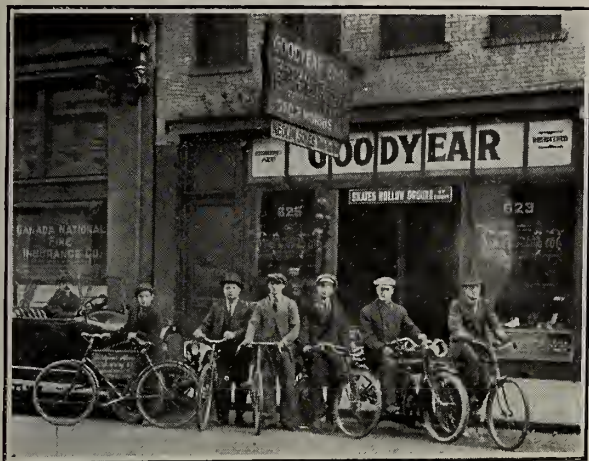
Exterior of Mr. Morris' store
