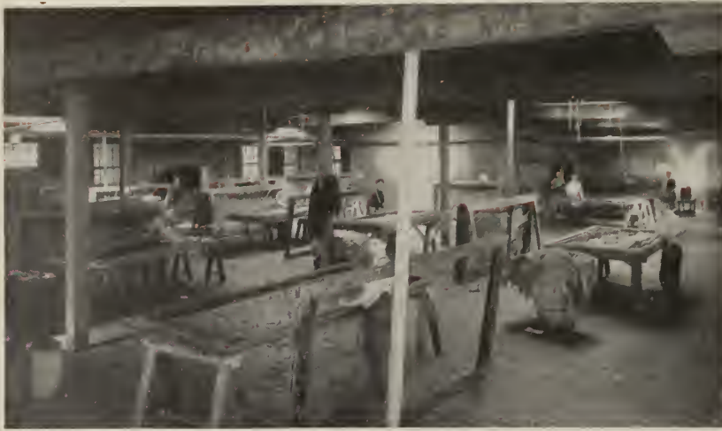
Section of Enamelling Factory, Producing 1,000 Sides Daily
