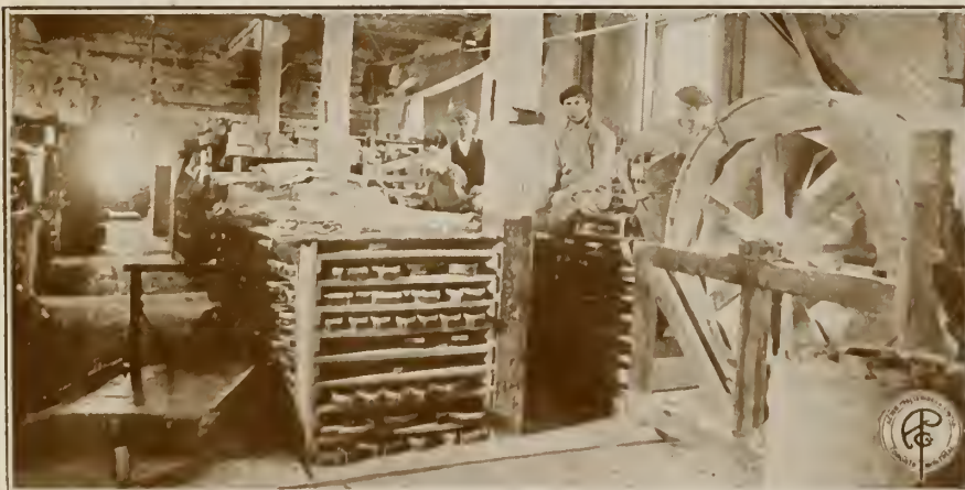
Inside Machine Cutting Room
