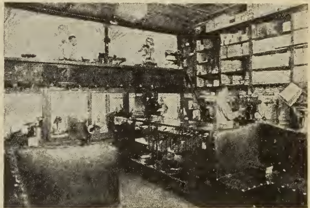
Showing location of repair department
