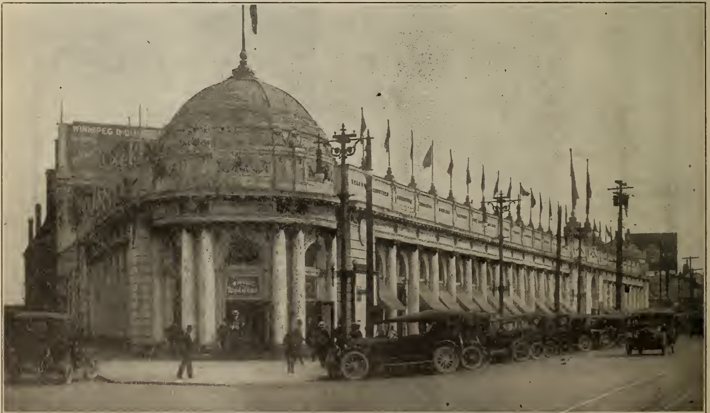
New Board of Trade Building, Winnipeg, Man. used as a permanent exhibit for Canadian industries.
