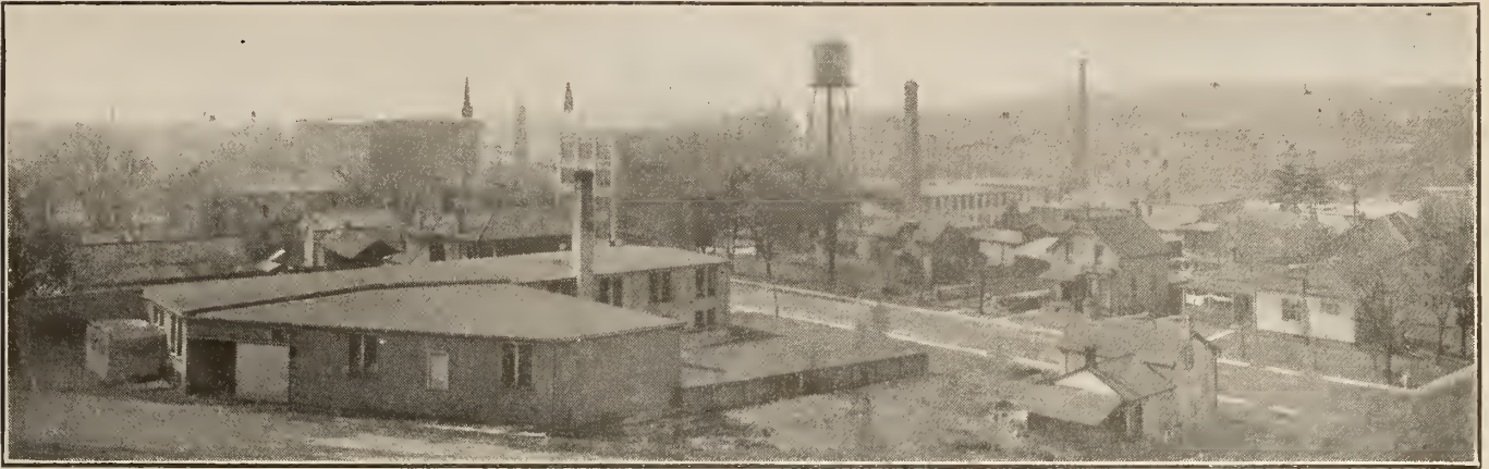
VIEW OF MANUFACTURING SECTION OF GALT.
