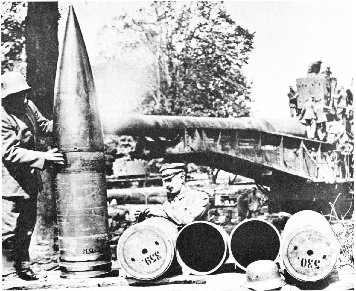
Artillery played a major role in WW I. Notice the tremendous size of the 380 mm shell fired by some German railroad guns
