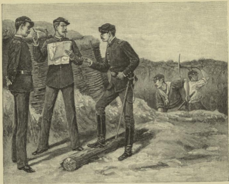
THE ENGINEER CORPS—INSTRUCTION IN FIELD FORTIFICATION.
