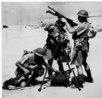
FIGURE 12.—Vickers gun on anti-aircraft mount.
