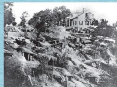
Earthworks at Vicksburg The siege of Vicksburg sees the besiegers and defenders both taking refuge in a system of trenches and dugouts little different from those of World War I half a century later. Starvation proves the Union army's strongest weapon.
