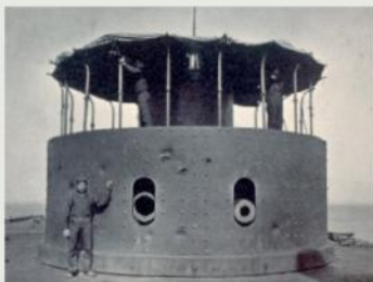
DAMAGED MONITOR TURRET
