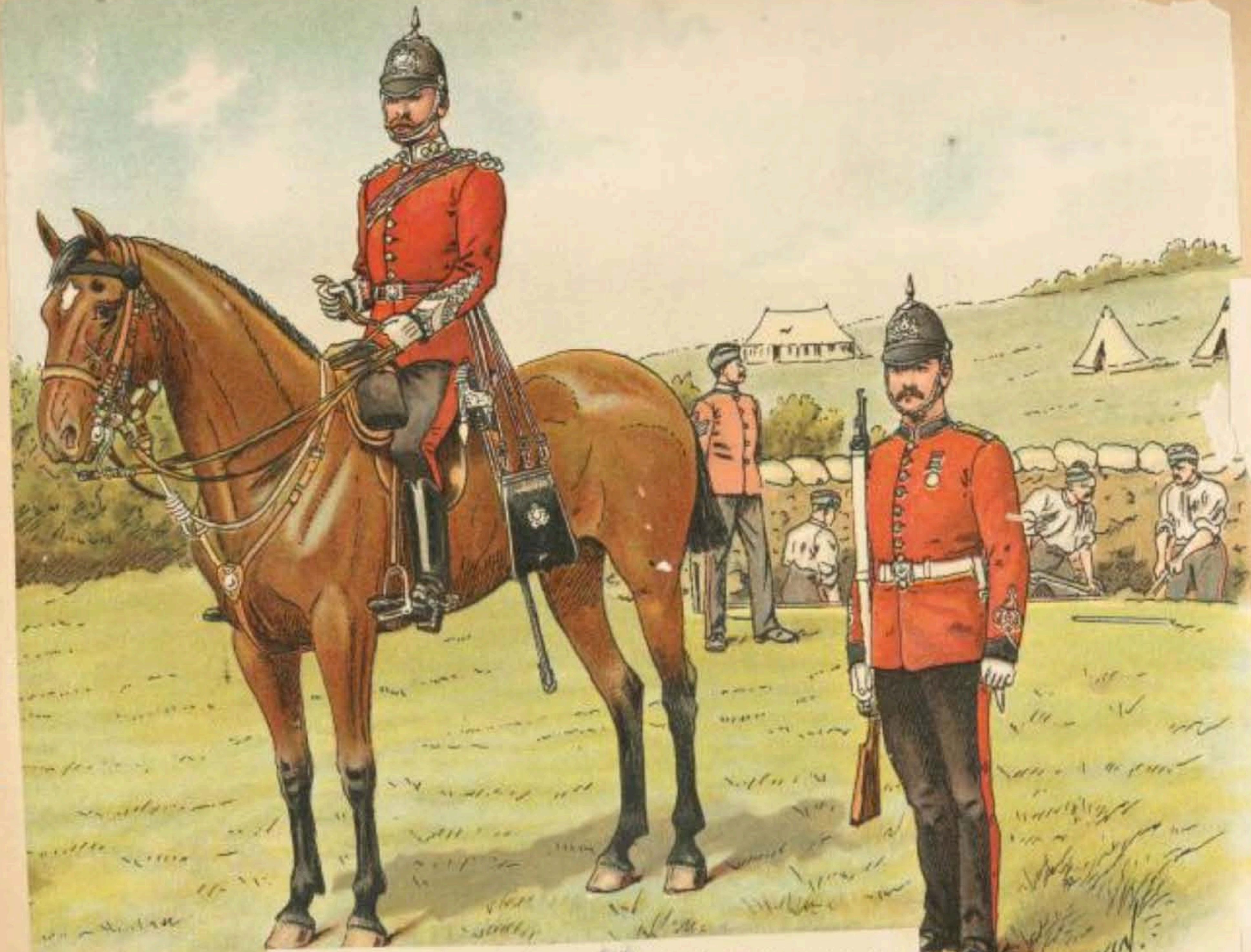
CONSTRUCTING SHELTER TRENCH. FIELD-OFFICER AND SAPPER, Review Order.
