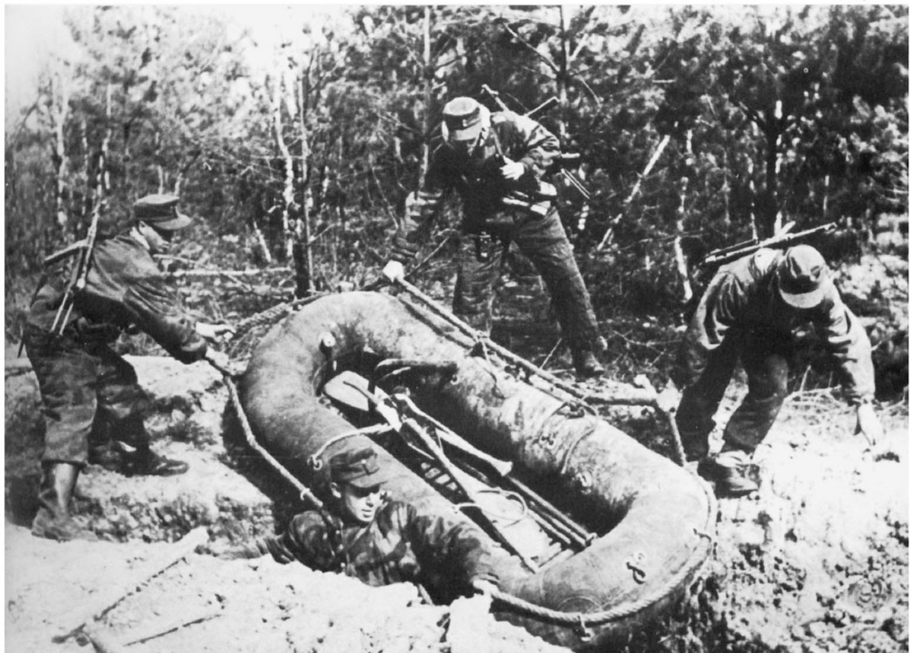
30 31. Soldiers quench their thirst with water trickling from a primitive wooden viaduct. 32. Large rubber, inflatable dinghies like this were used as floating pontoons for bridge building and for transporting troops during
