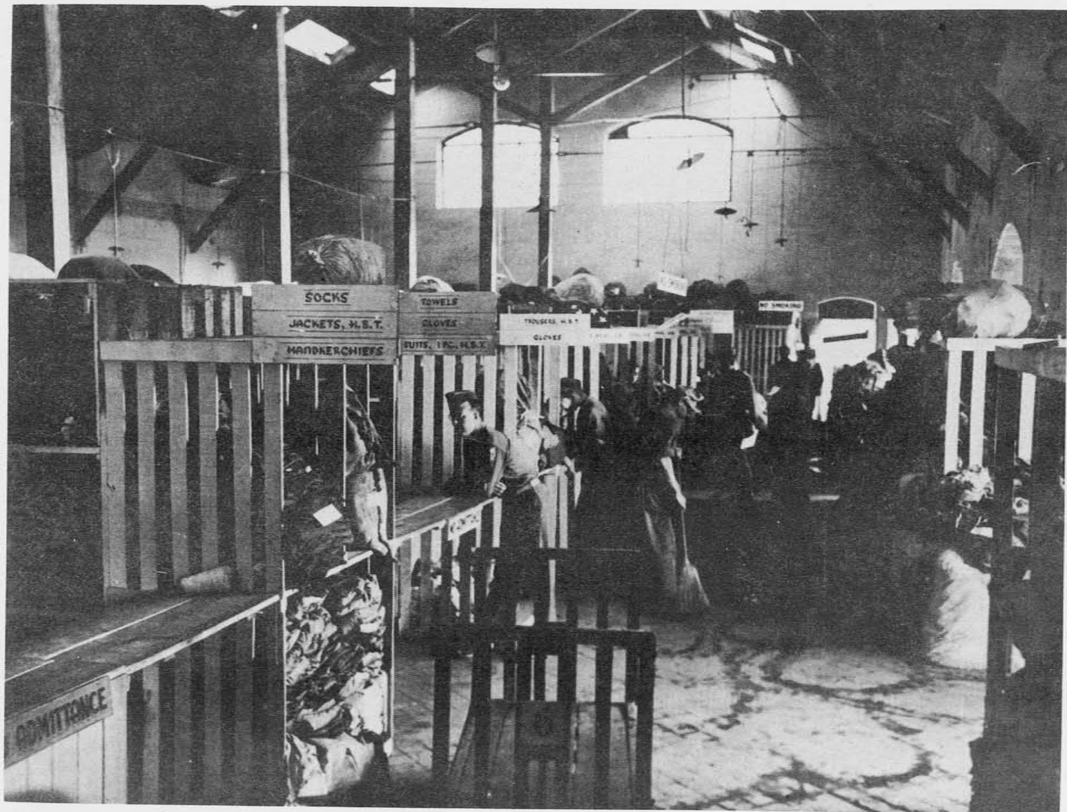
Figure 21.—Inside View of Clothing Warehouse at Reims.
