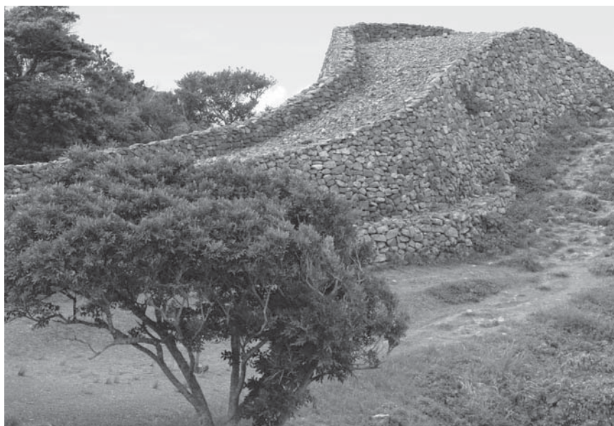
The graceful sweep of the walls of the gusuku of Nakijin. Here the walls follow the contour of the hill. The walls are made of limestone.
