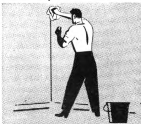
First clean the corners and then the bulkheads.
