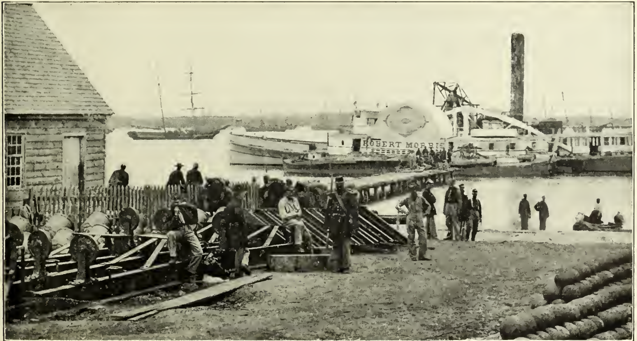
LOADING THE TRANSPORTS
