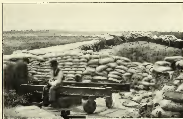
THE MISSING RIFLE. (Extensive sand-bag fortifications of the Confederates at Yorktown.) The shells and carriage were left behind by the Confederates, but the rifled gun to which they belonged was taken along in the retreat. Such pieces as they could not remove they spiked.
