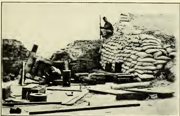
ANOTHER VOICELESS GUN. (Confederate ramparts southeast of Yorktown.) A 32-pounder Navy gun which had burst, wrecking its embrasure. The Federal soldier seated on the sand-bags is on guard-duty to prevent camp-followers from looting the vacant fort.
