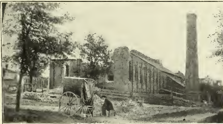
RUINS OF STATE ARMORY, COLUMBIA, 1865
