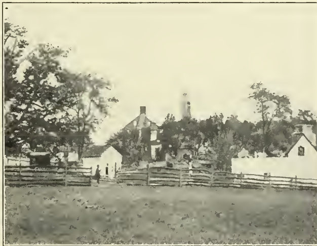
RUIN OF MUMMA'S HOUSE, ANTIETAM
