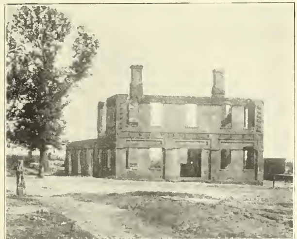
THE SOUTH CAROLINA RAILROAD OFFICES
