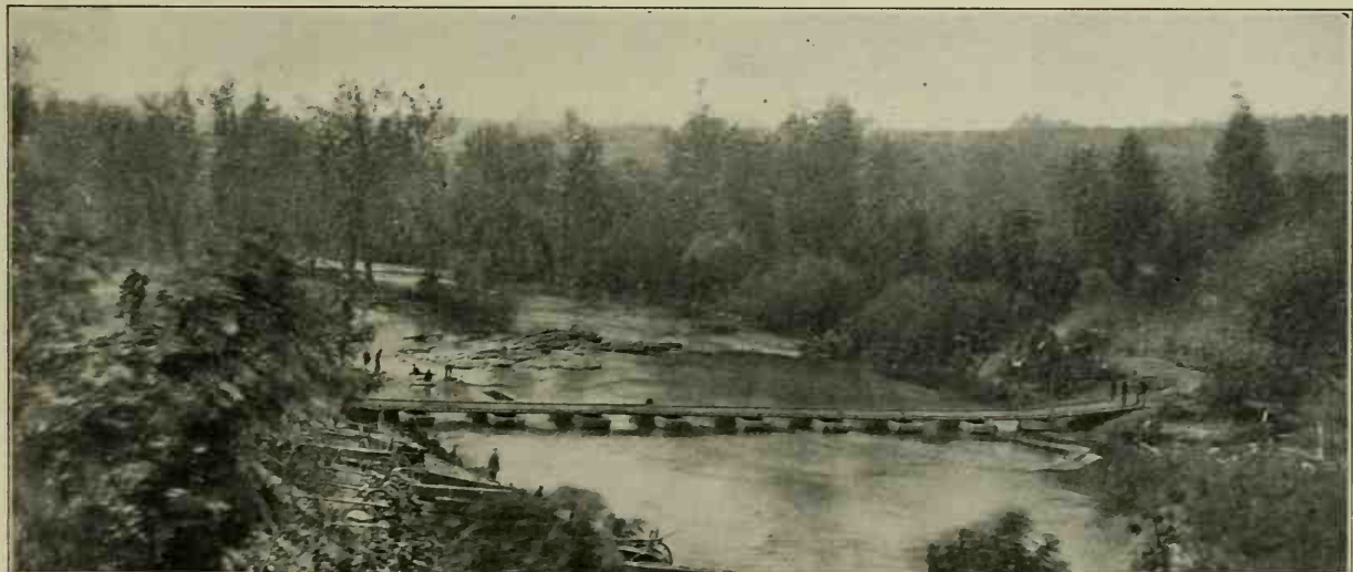
THE BRIDGE FROM UPSTREAM, JERICHO MILLS
