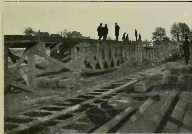
TESTING A "SHAD-BELLY" BRIDGE
