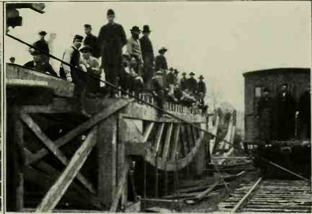
LOADING A BRIDGE TO TEST IT
