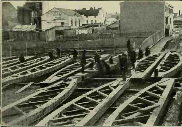
BUILDING PORTABLE BRIDGE-TRUSSES
