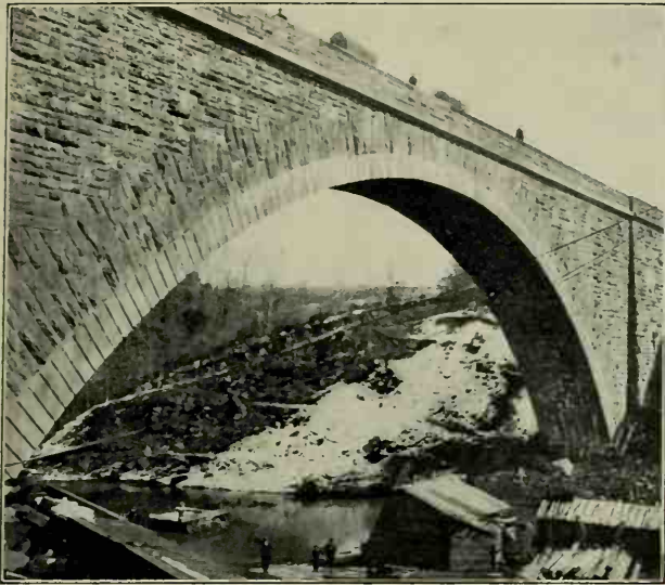
UNION ARCH OF THE WASHINGTON AQUEDUCT
