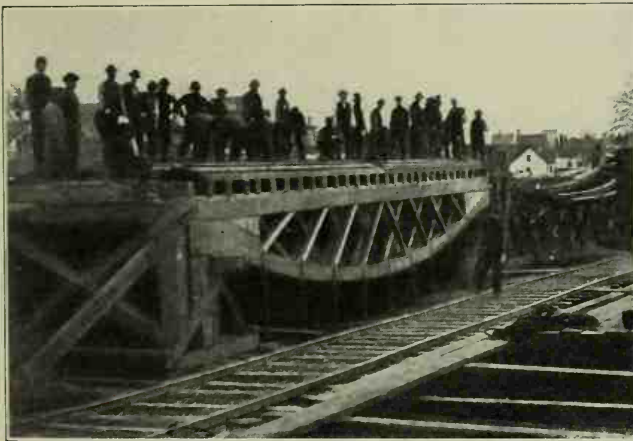
EXPERIMENTS WITH BOARD TRUSSES
